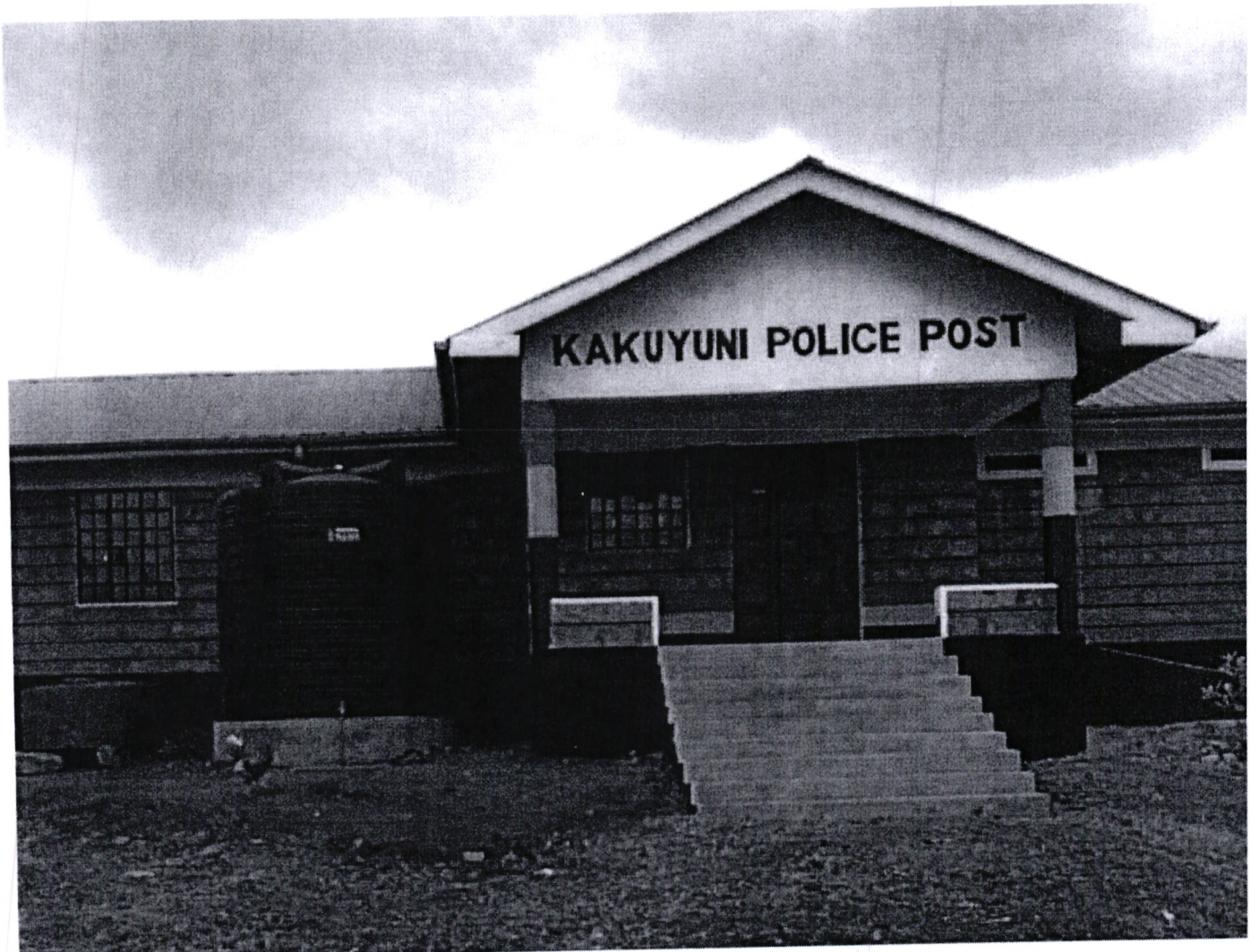
• Fig.3 Kakuyuni Police Post Completion -Kshs. 3,741,720.00
