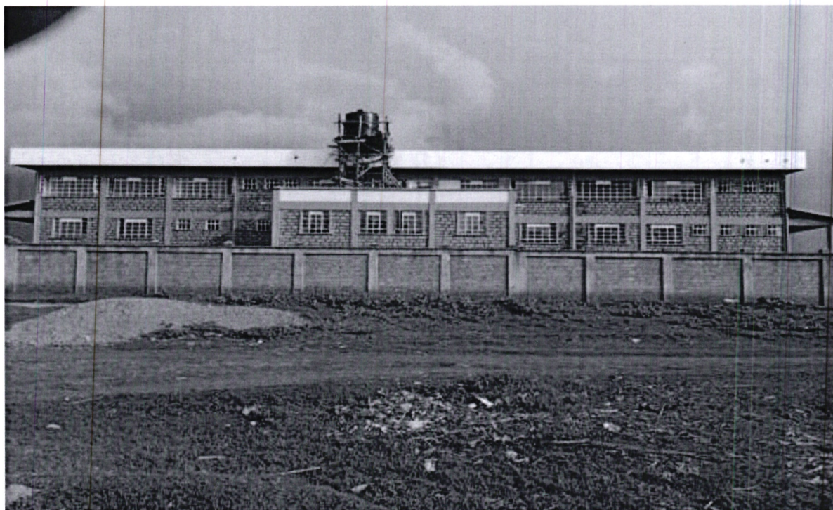
Manga Stadium (Muilt Year Project)
