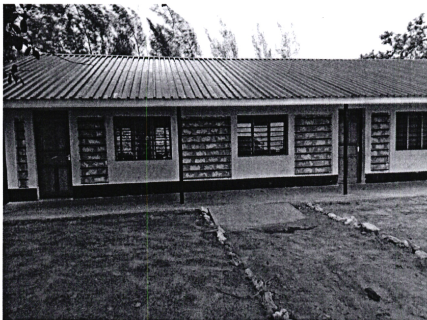
Kanana Genesis Primary School-2 No. Classrooms
