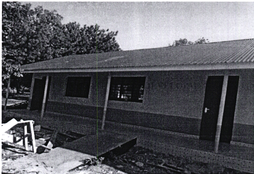
Mwalewa Primary School – 2No. Classrooms
