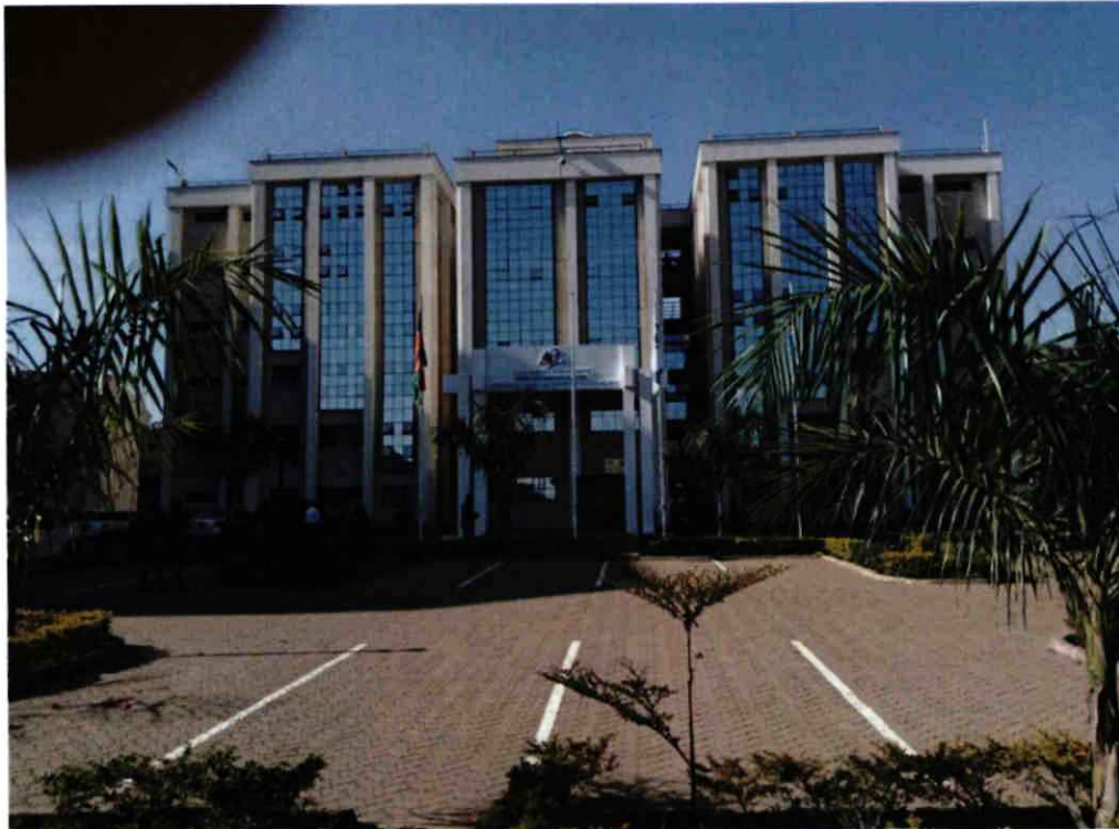
Administration and Lecture Halls Block
