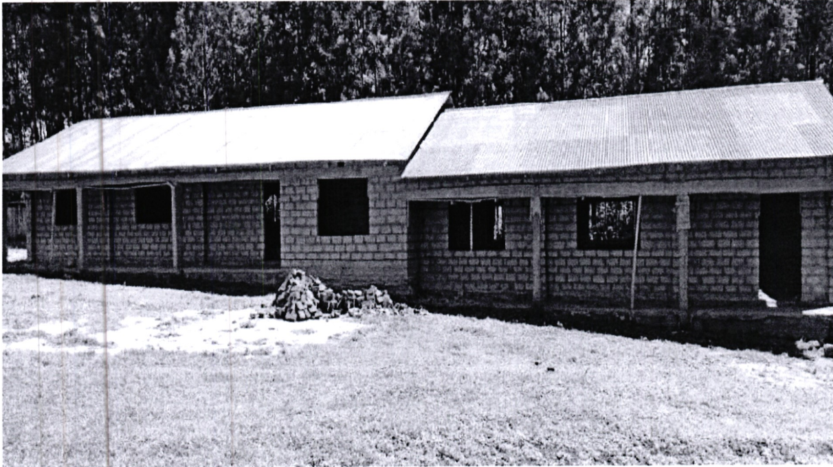
Ongoing construction of twin lab at Nakoba Friends Secondary School
