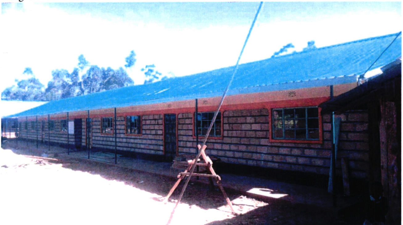
DEB Ontulili Primary School construction of 4 classrooms FY 2019/2020
