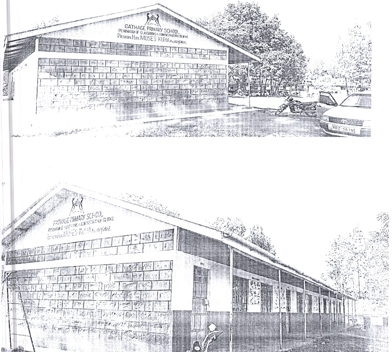
Fig 1.1 Gathage Primary School – Renovation of classrooms and administration block
