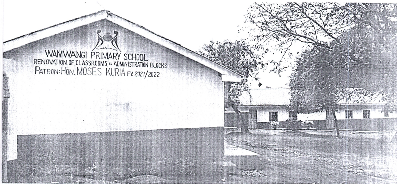
Fig 1.2 - Wamwangi primary school- Renovation of classrooms and administration block
