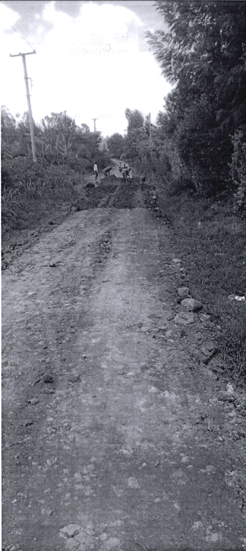
Access road repairs in Embu Zone
