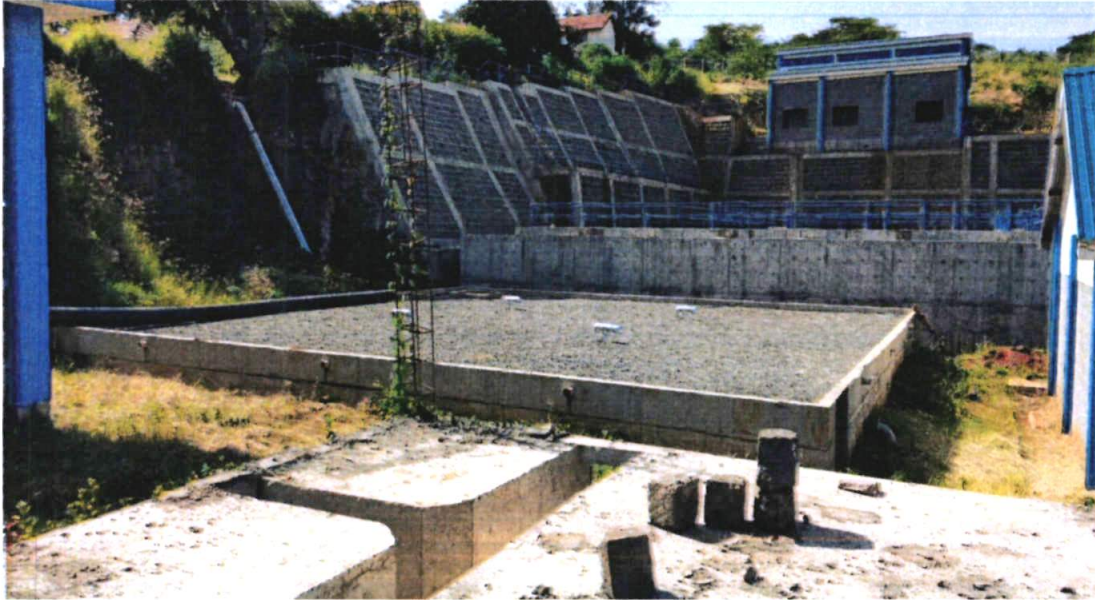
Figure 1: Completed Treatment plant at Machakos Water Project
