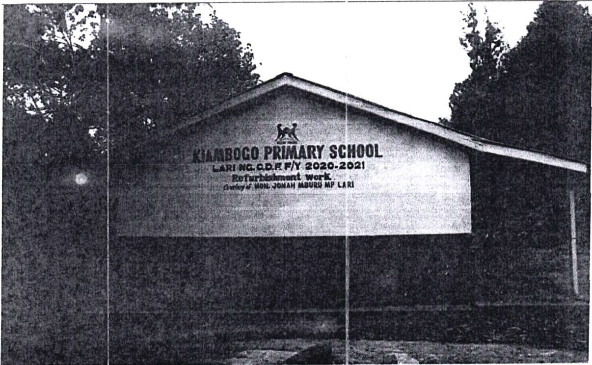
KIAMBOGO PRIMARY SCHOOL RENOVATION OF THE WHOLE SCHOOL
