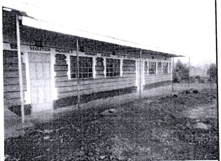
Segutioi Ngariet Pri School-Construction of 2 classrooms-Kiptororo Ward
