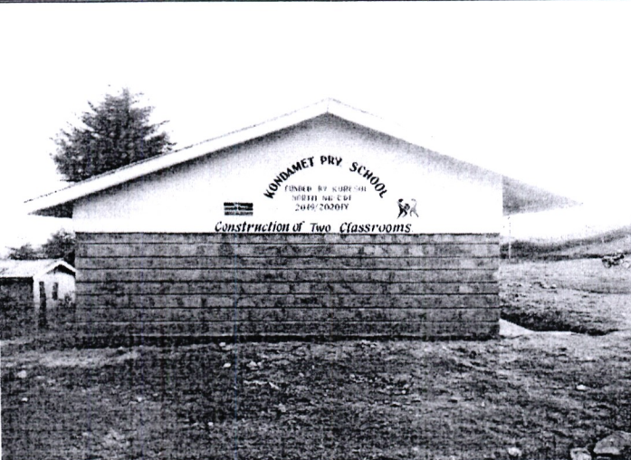
Kondamet Pri School-Construction of two Classrooms-Nyota Ward
