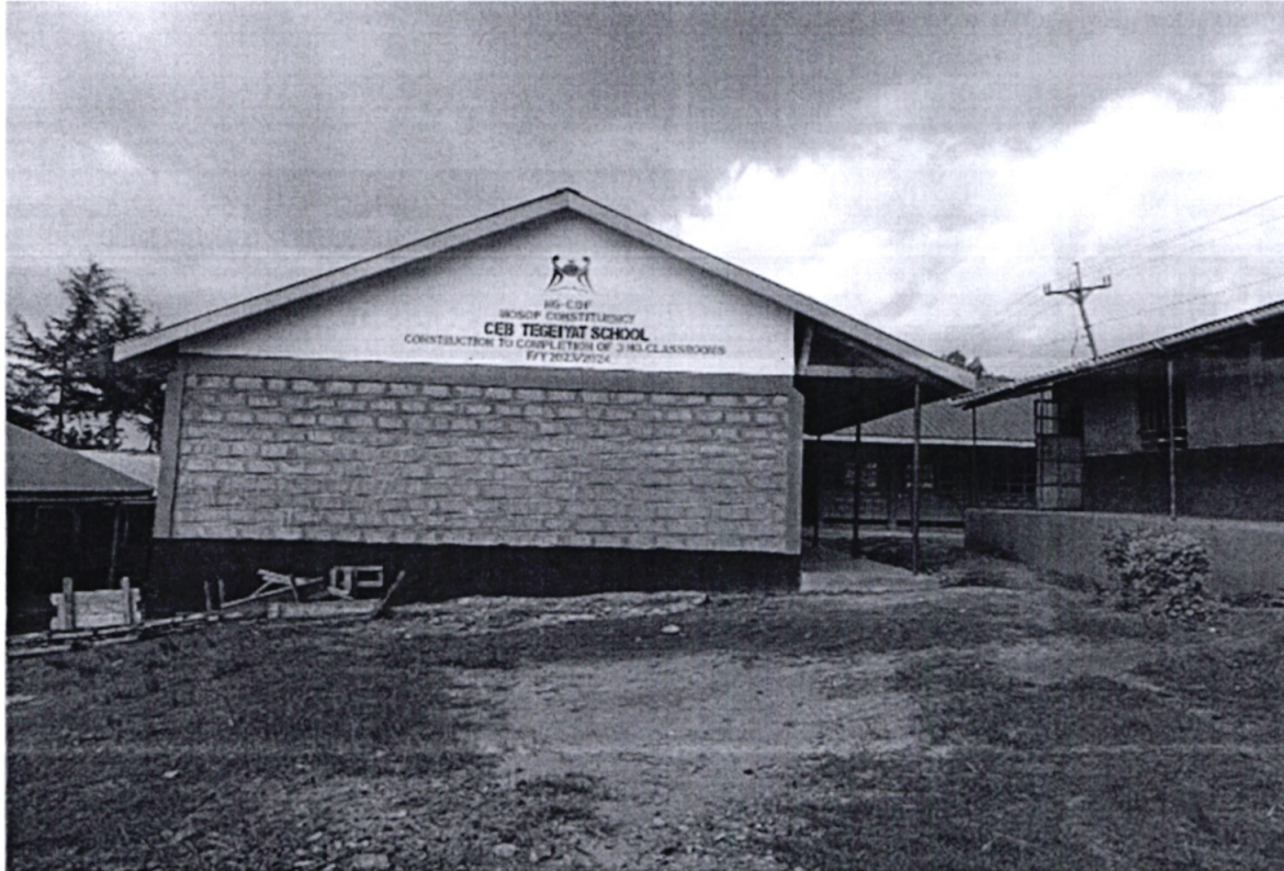
Fig 2: Tegeiyat Primary School-Construction to completion of a 3 No Classrooms
