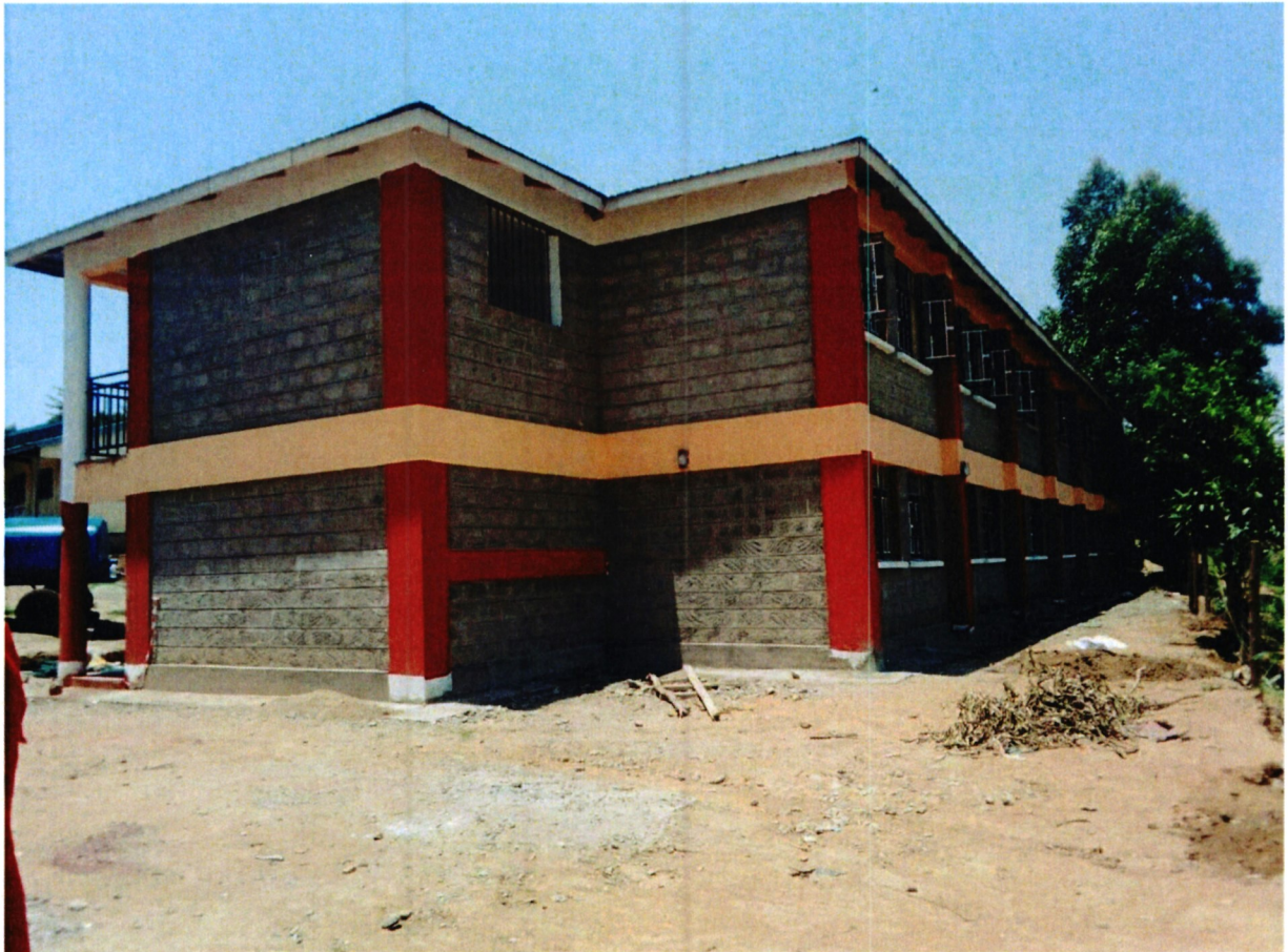
Picture 3- Chengoli Primary School Webuye West- Construction of 6 Classrooms
