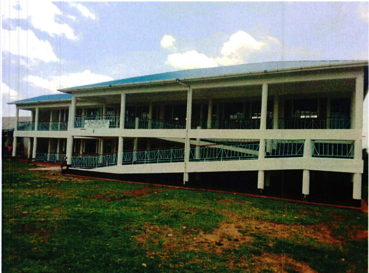
Picture- Lugulu day Secondary School Webuye West- Six classrooms storey block with ramp
