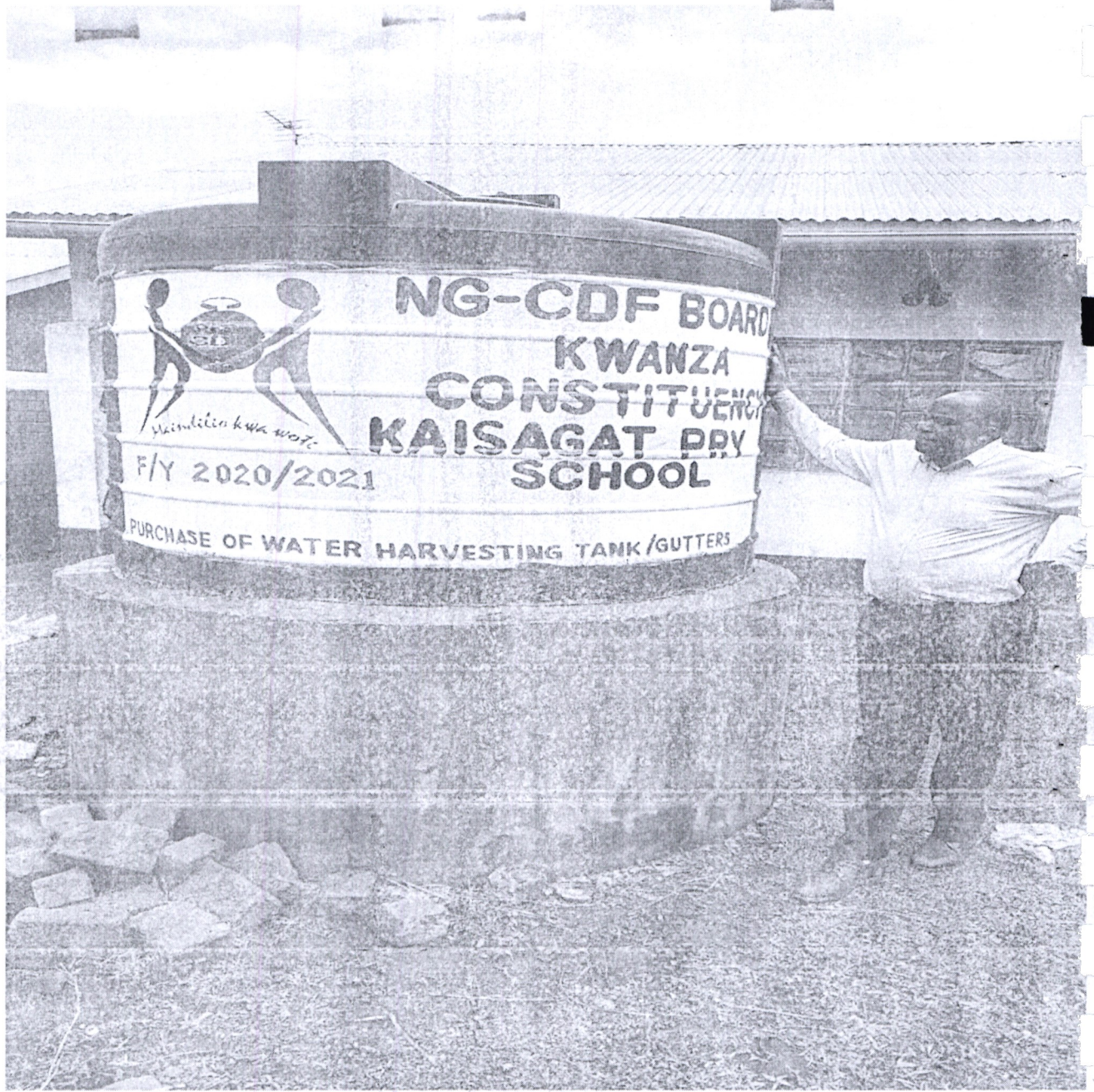
KAISAGAT PRIMARY SCHOOL-PURCHASE AND INSTALLATION OF 10,000 LTRS WATER TANK AND GUTTERS
