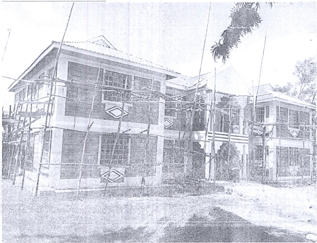
BIDII DIVISIONAL HEADQUATERS, CONSTRUCTION OF ACC'S OFFICES-ONGOING
