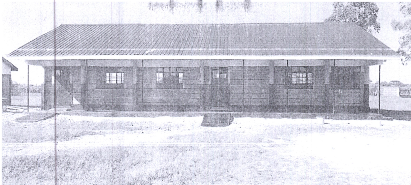
NDALALA PRIMARY SCHOOL, CONSTRUCTION OF TWO CLASSROOM-COMLETE
