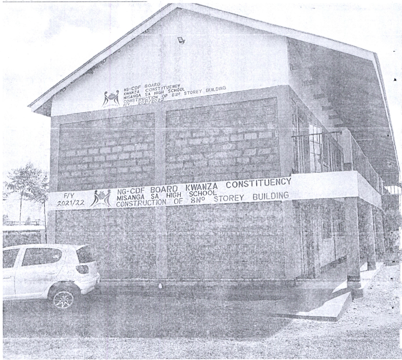
MISANGA S.A SEC.SCHOOL, CONSTRUCTION OF A STOREY TUITION BLOCK OF EIGHT CLASSROOMS-COMPLETE.
