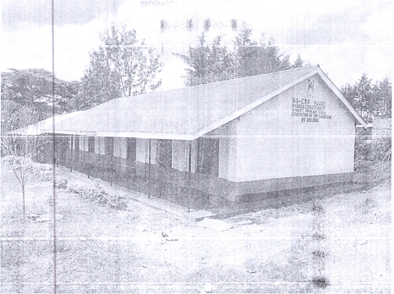
AINASIT PRIMARY SCHOOL, RENOVATION OF TWO CLASSROOM- COMPLETE
