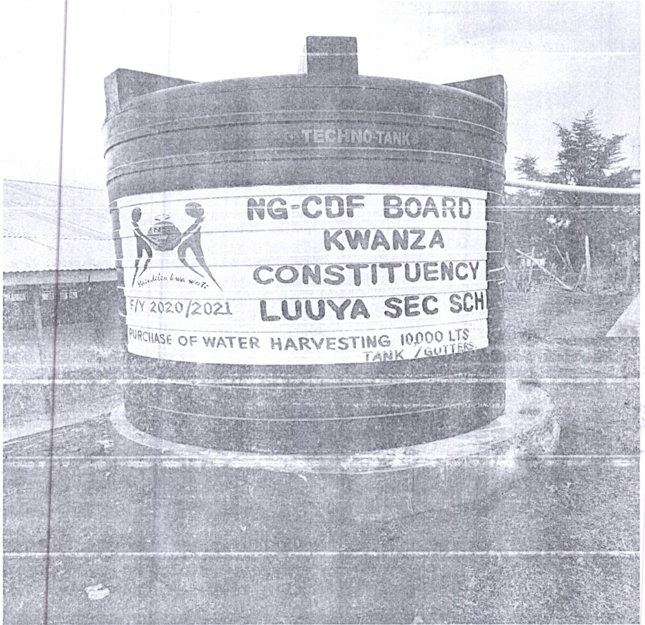
LUUYA SECONDARY- PURCHASE AND INSTALLATION OF 10,000 LTRS WATER TANK AND GUTTERS-COMLETE
