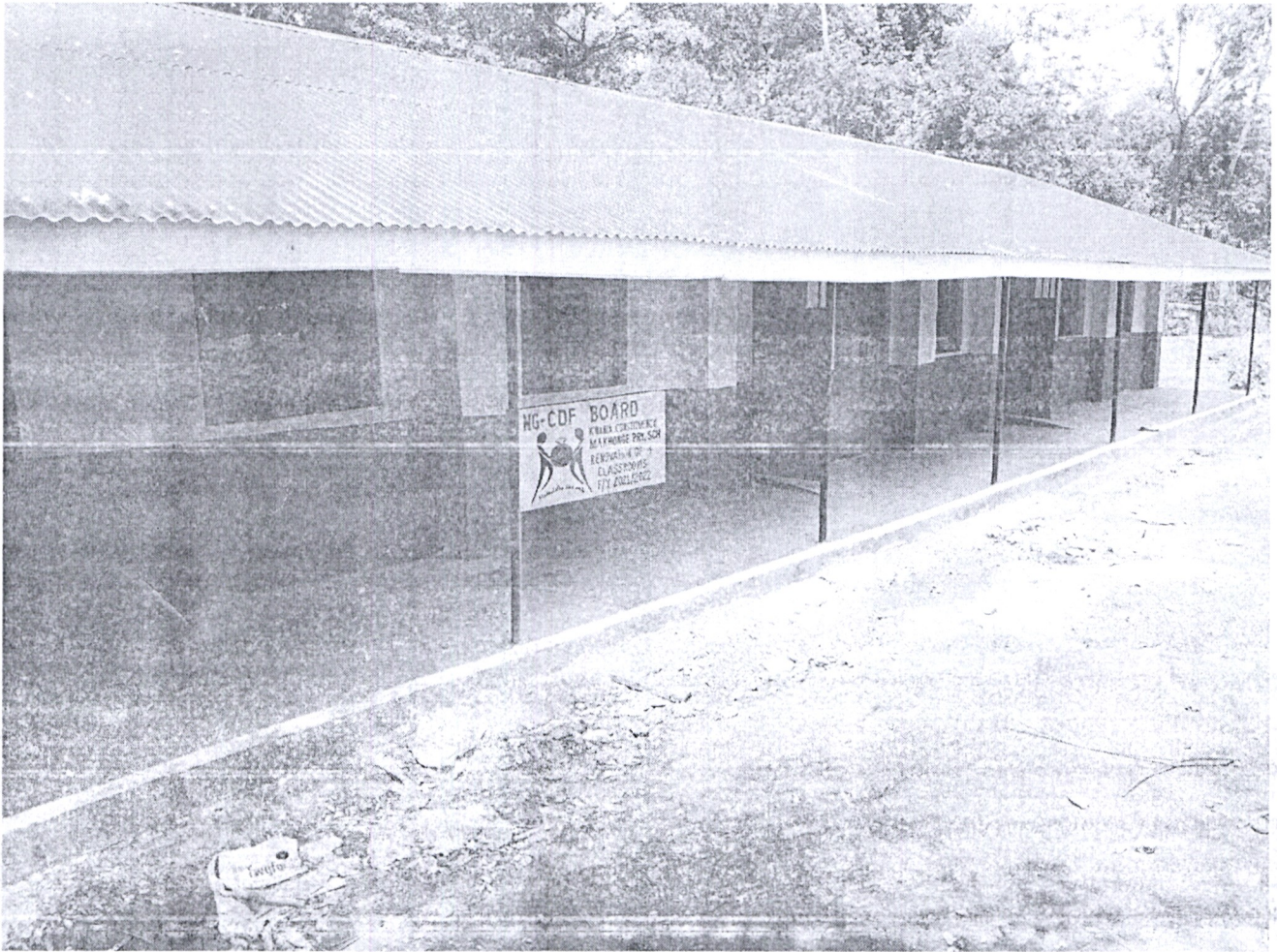
MAKHONGE PRI.SCHOOL, RENOVATION OF FOUR CLASSROOMS-COMplete
