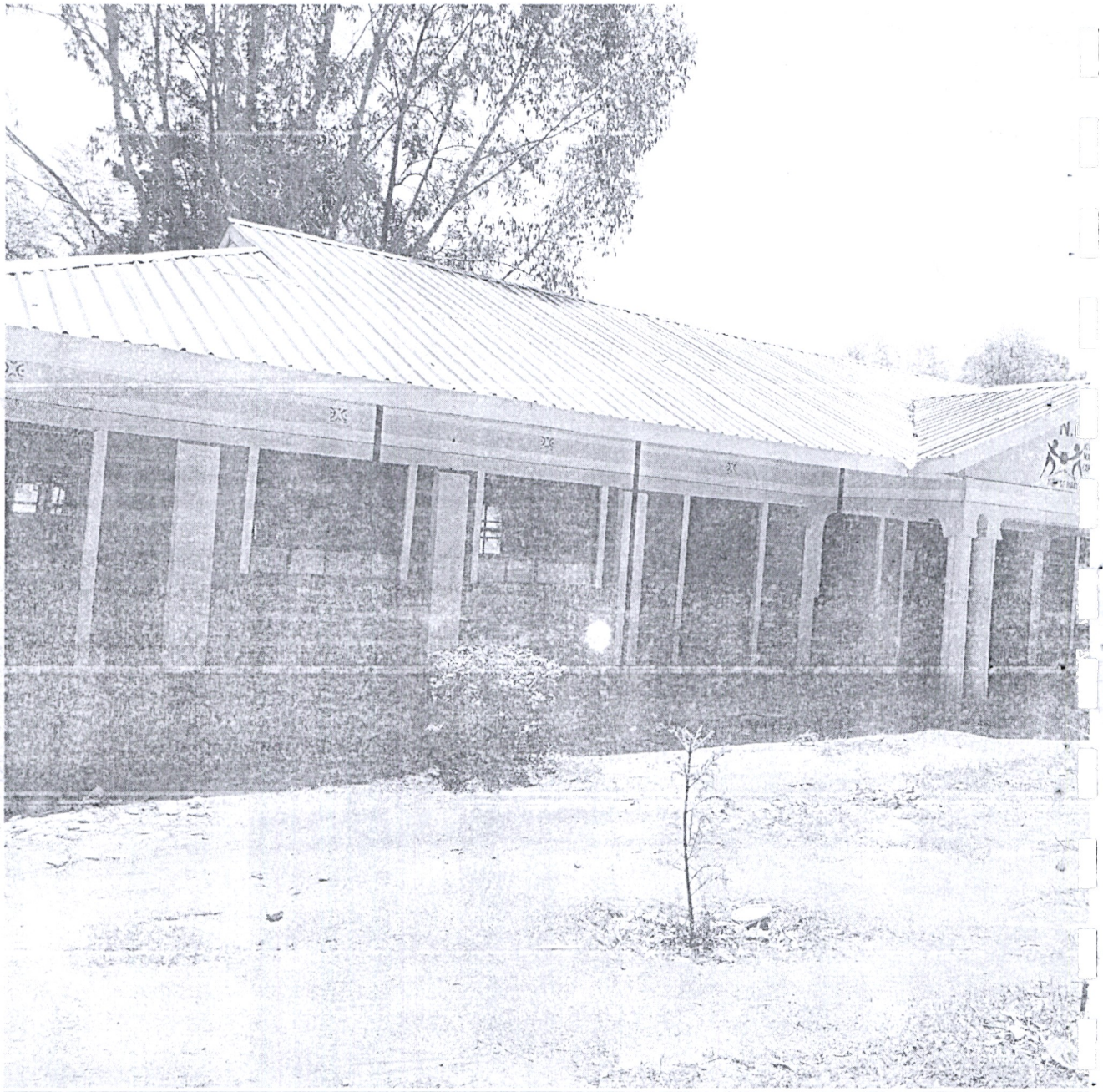
NAMANJALALA SECONDARY SCHOOL, CONSTRUCTION OF A TWIN LABORATORY- COMPLETE.
