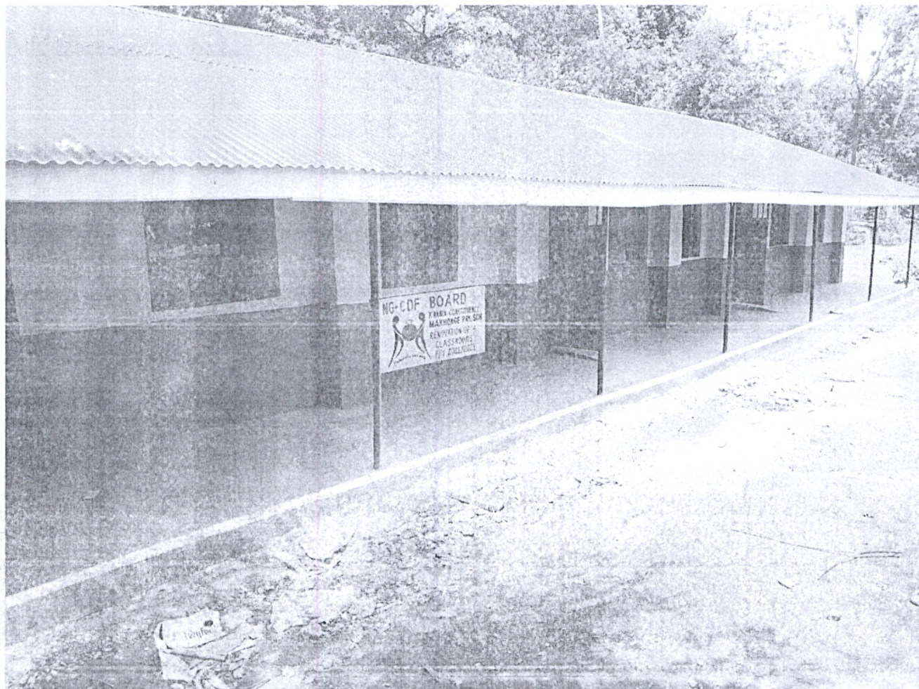
MAKHONGE PRI.SCHOOL, RENOVATION OF FOUR CLASSROOMS-COMPLETE
