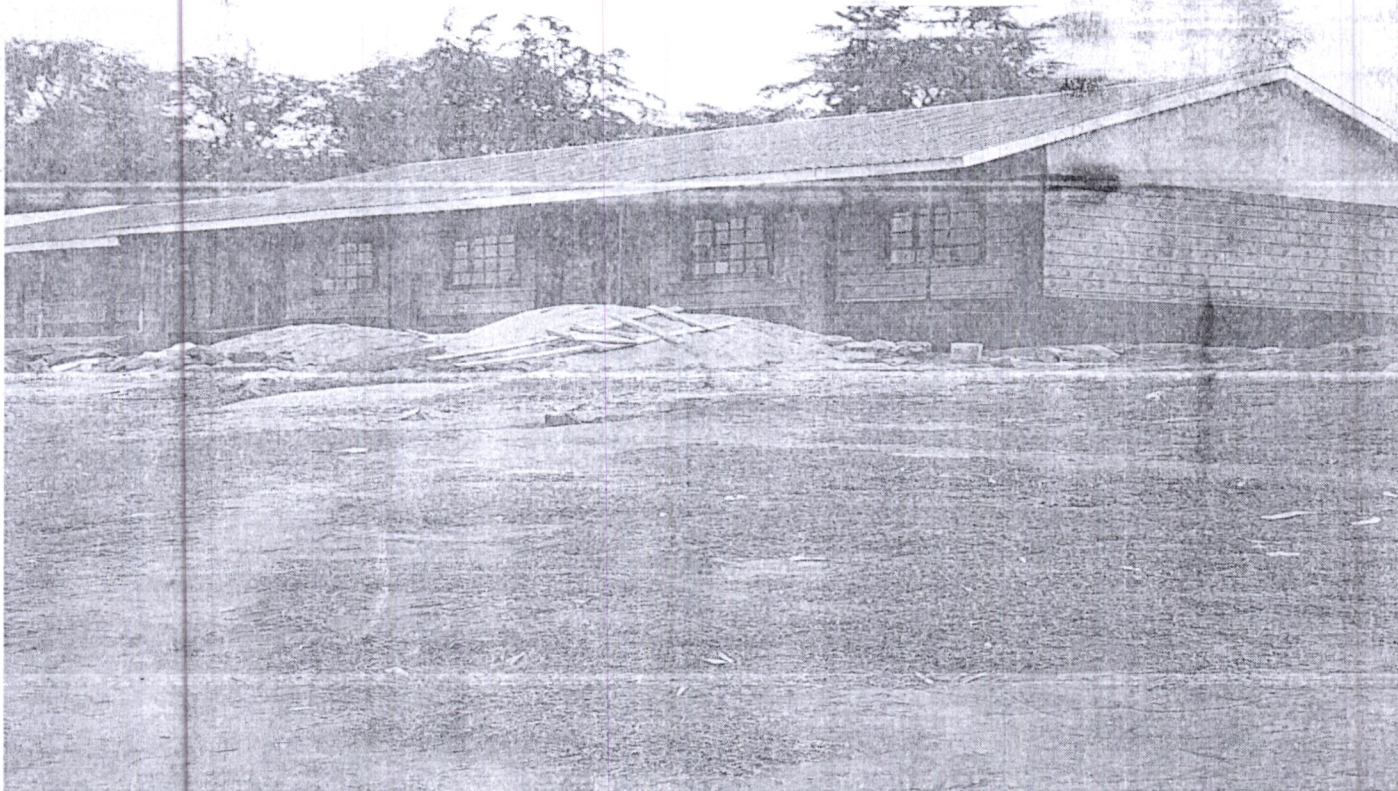
WATER SUPPLY PRIMARY, CONSTRUCTION OF TWO CLASSROOMS-COMLETE
