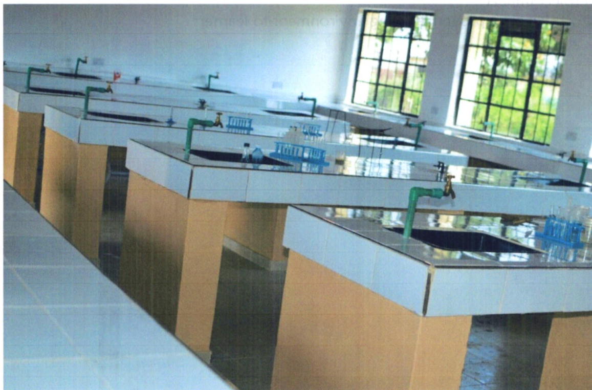
Figure 6: Construction Of 60 Pax Science Laboratory At St Anthony Pala Kobong' Secondary School
