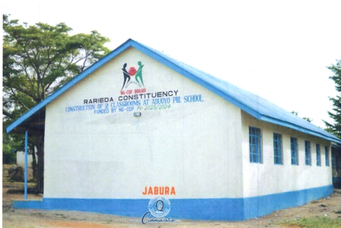
Figure 5: Construction of 2 classrooms at Aduoyo Primary School
