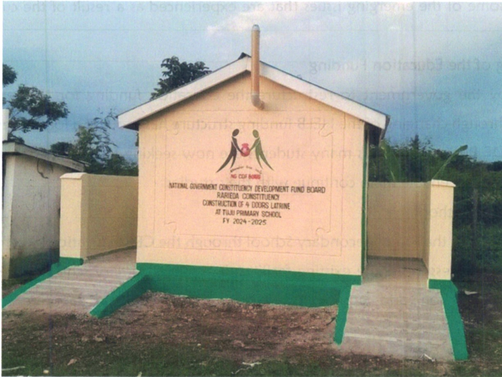
Figure 2: Construction of 4 No door pit latrine at Tuju Primary School
