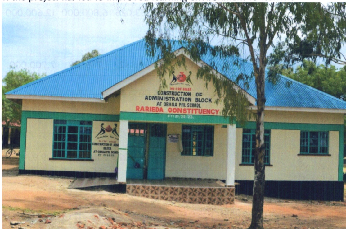
Figure 4: Construction of Admin Block at Obaga Primary School
