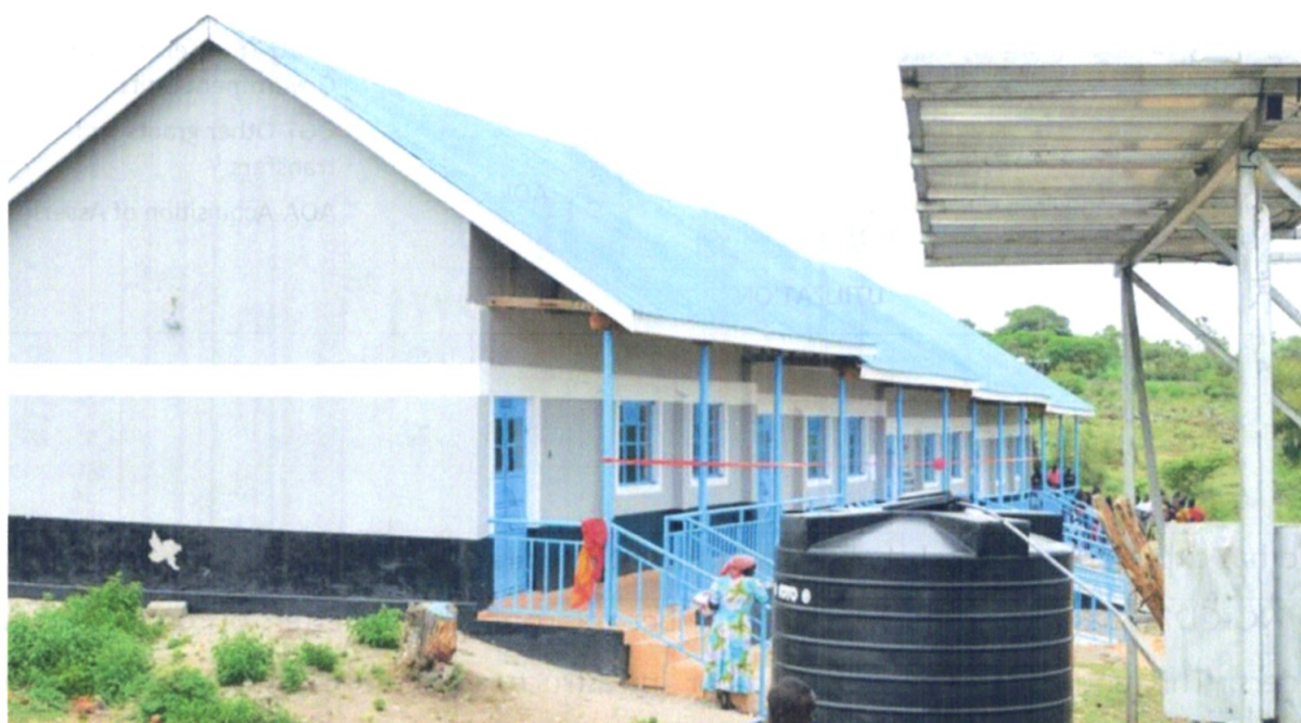
Figure 1: Construction of 4 Classrooms at Osewre Primary School.
