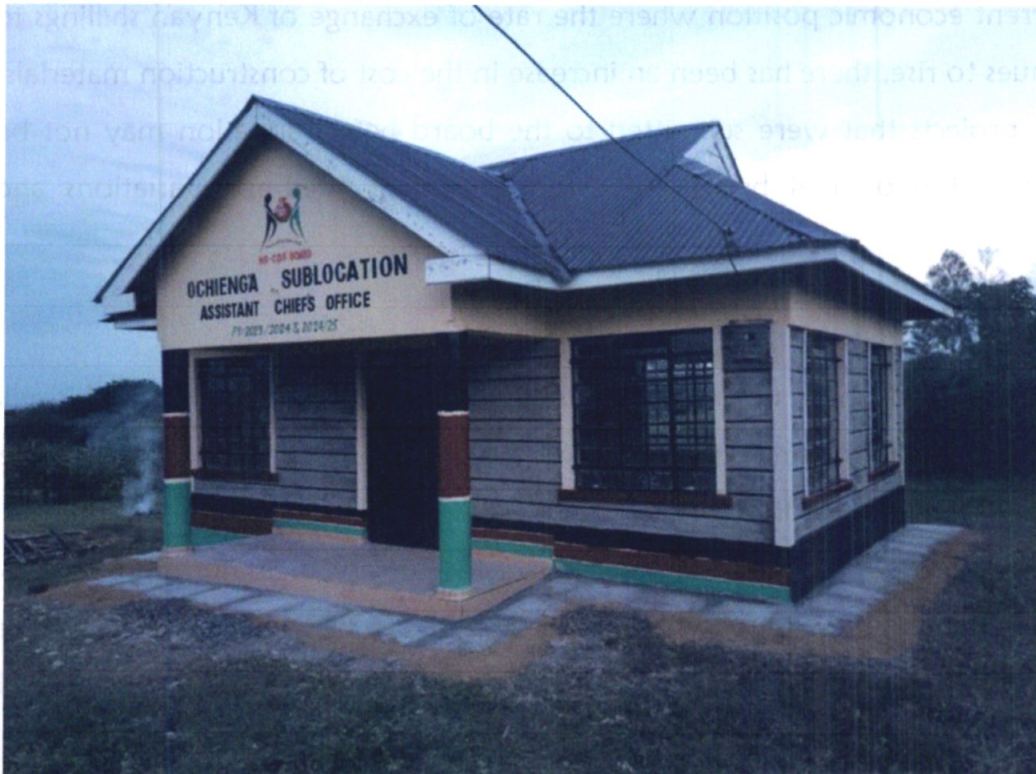
Figure 3: Construction of Ochieng'a Sublocation Assistant Chief's Office
