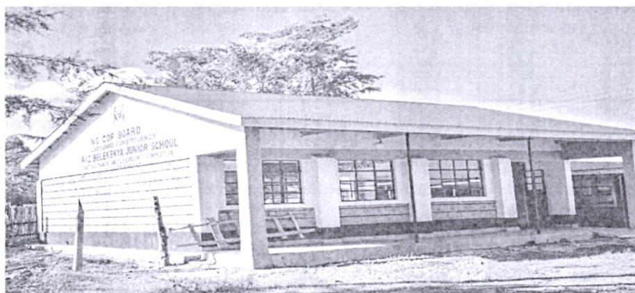
Belekenya Junior School- Construction to completion of 1 Classroom
