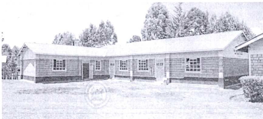
AIC Cheptwolio Secondary school- Completion of Dining Hall
