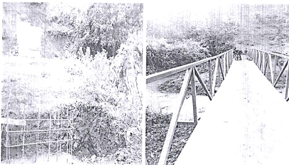
Ongoing footbridge construction works, Complete steel fabricated footbridge Chepseon Ward
