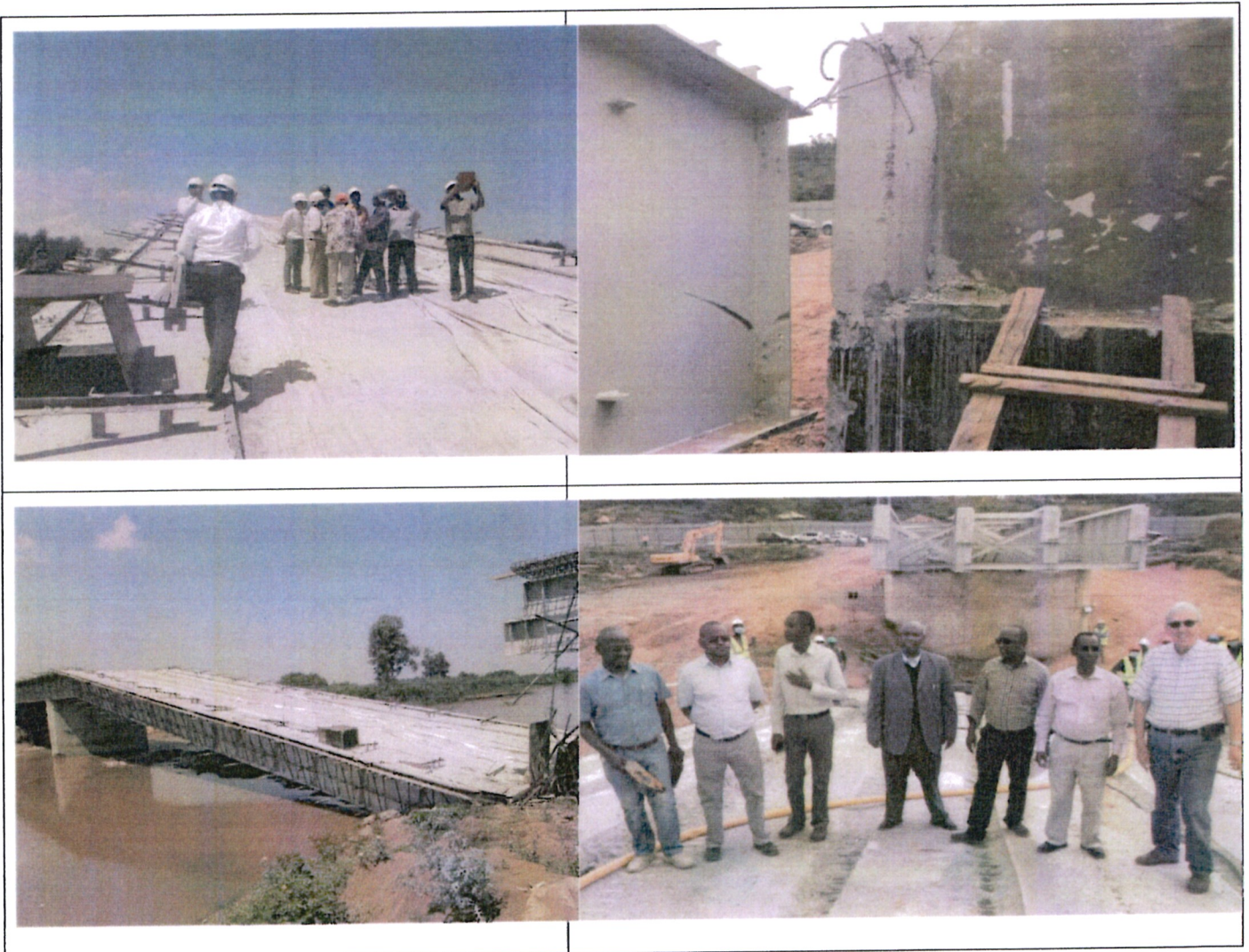
Investigations into collapse of Sigiri Bridge
