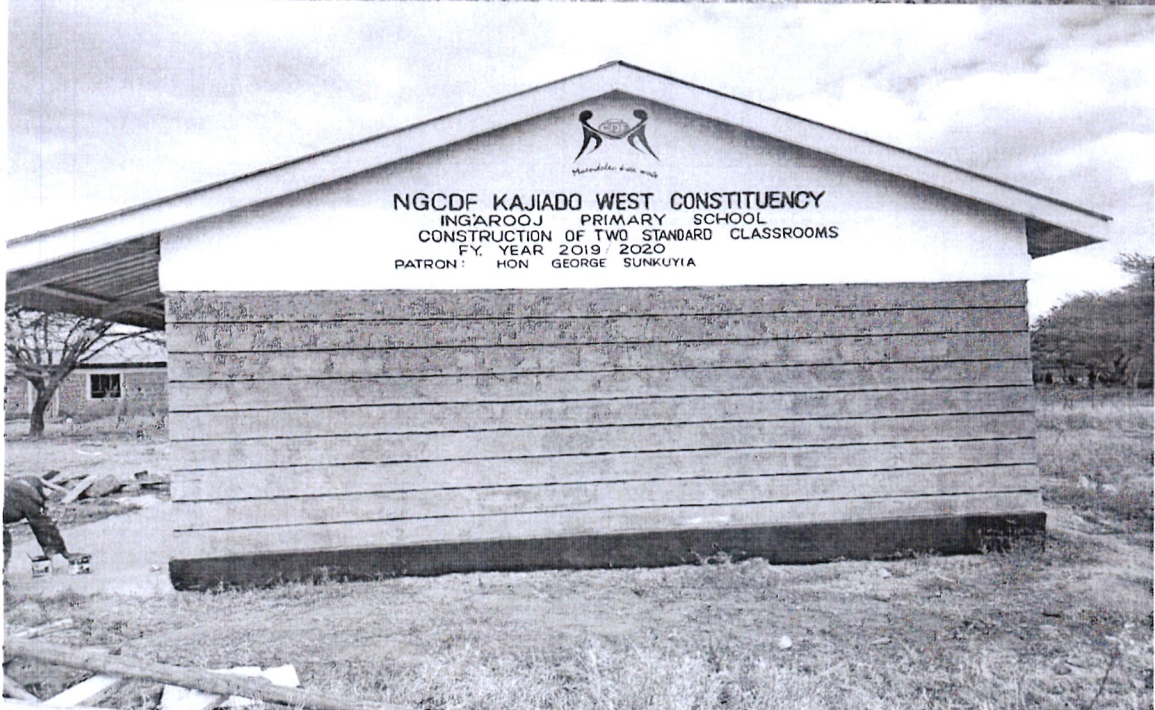
2 NO. CLASSROOMS AT ILNGAROJ PRIMARY SCHOOL FUNDED BY NGCDF KAJIADO WEST FY 2019/20.
