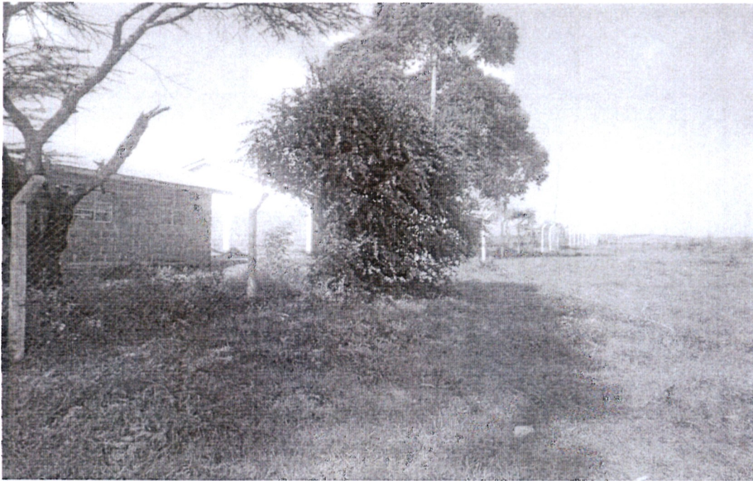
COMPLETED OLCHORO-ONYORI PRIMARY SCHOOL AFENCING AND GATE FUNDED BY NGCDF KAJIADO WEST 2018/19.
