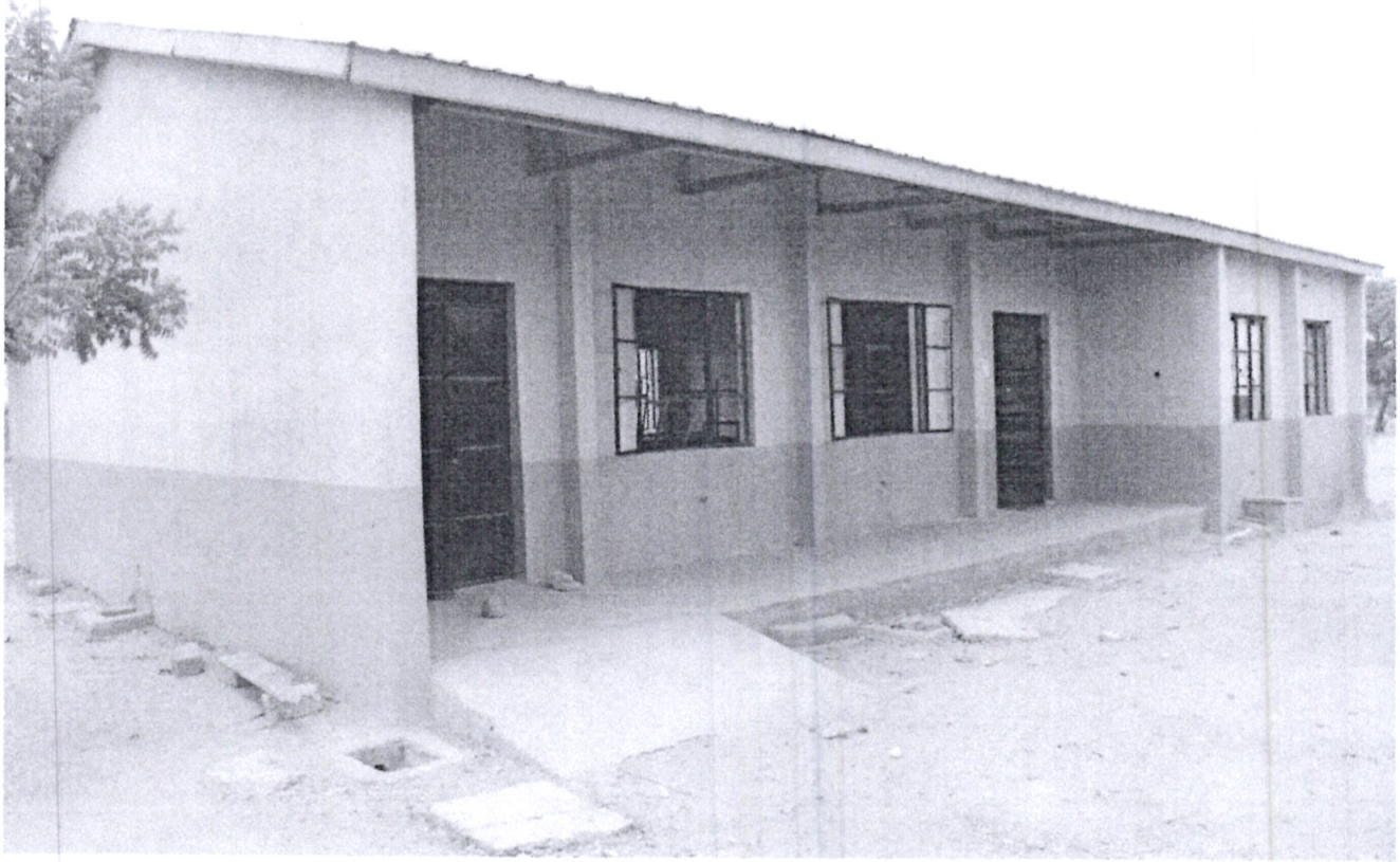
CHANANI SECONDARY SCHOOL LABORATORY
