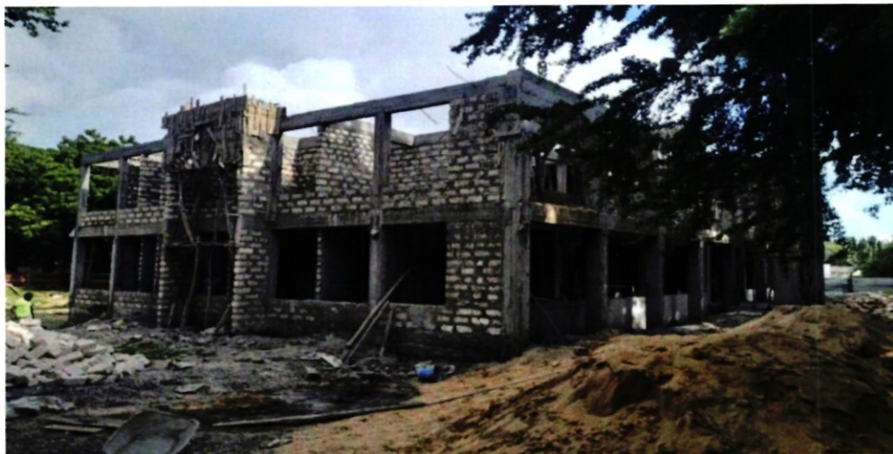
Picture 2: Ongoing Construction of Kilifi TSC County Office
