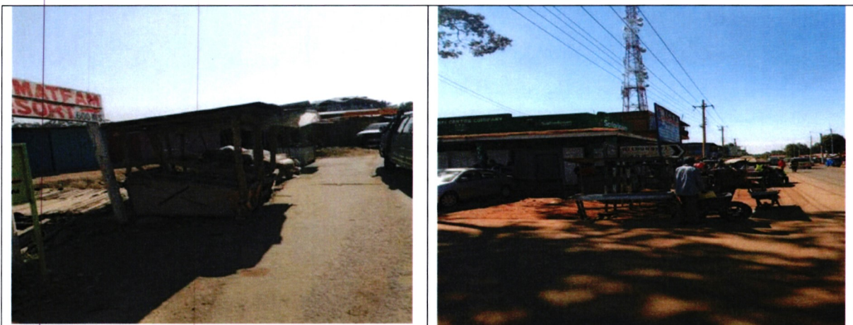
Figure 5: Encroachment along Roads
