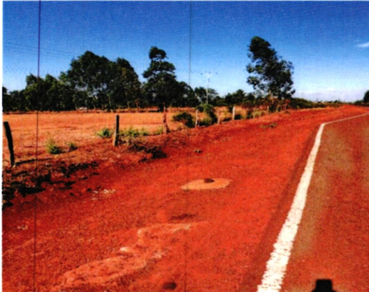
Figure 8: Vandalised Road Furniture
