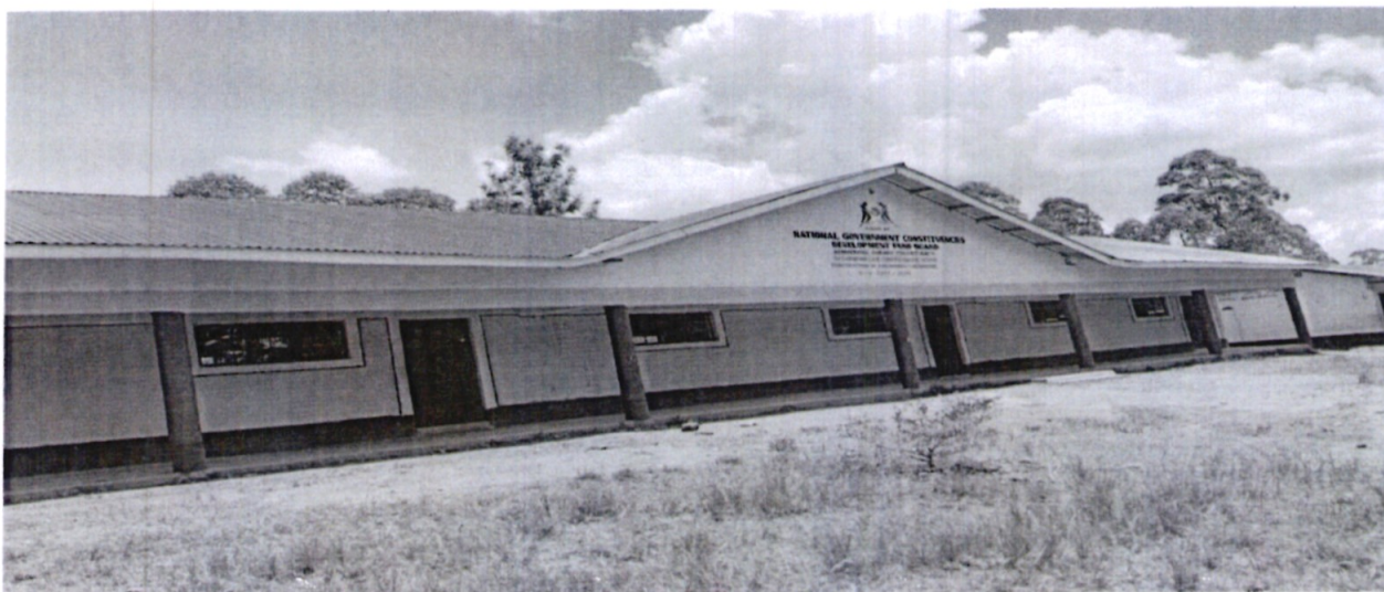
Gesabakwa SDA Comprehensive School : Construction to completion of 3 classrooms
