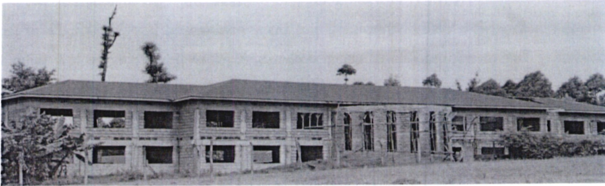
Kenyoro PAG School: Construction of 8 No classrooms on a 1 storey building.
