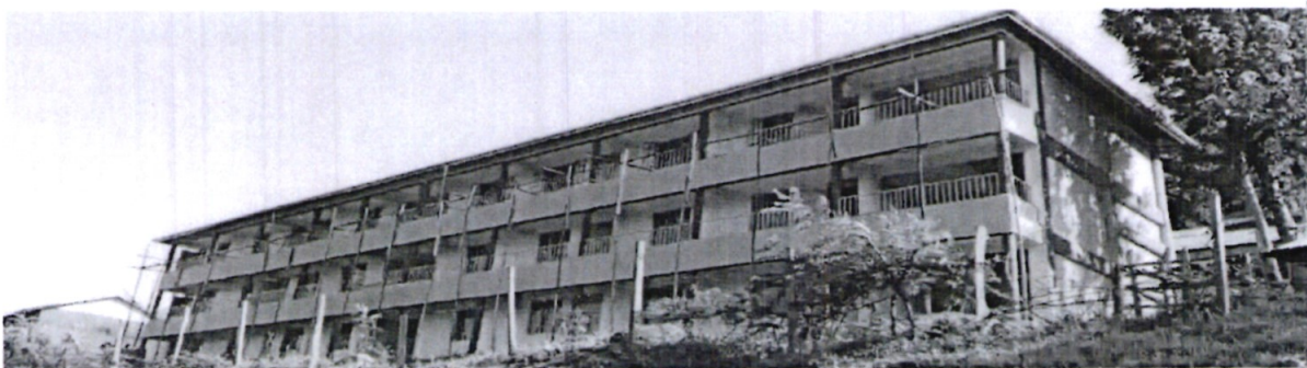
Nyakorere Primary School: Construction of 12 No classrooms on a 2 storey building.
