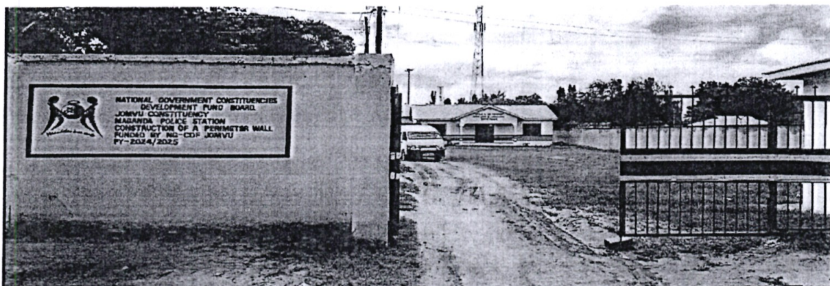
Maganda Police Station – construction of perimeter wall
