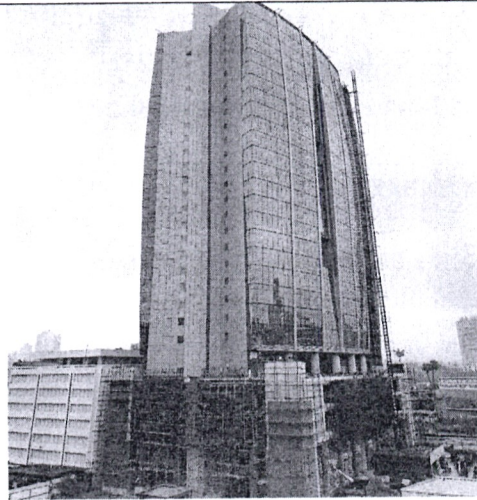
Multi Storey Office Block
