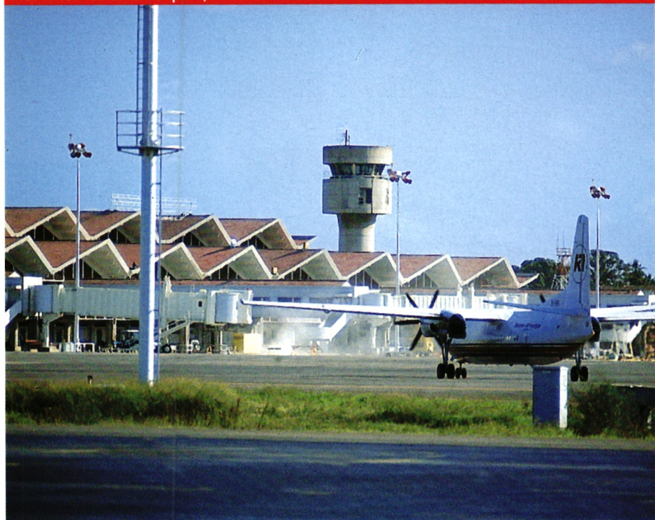
Moi International Airport, Mombasa after rehabilitation.
