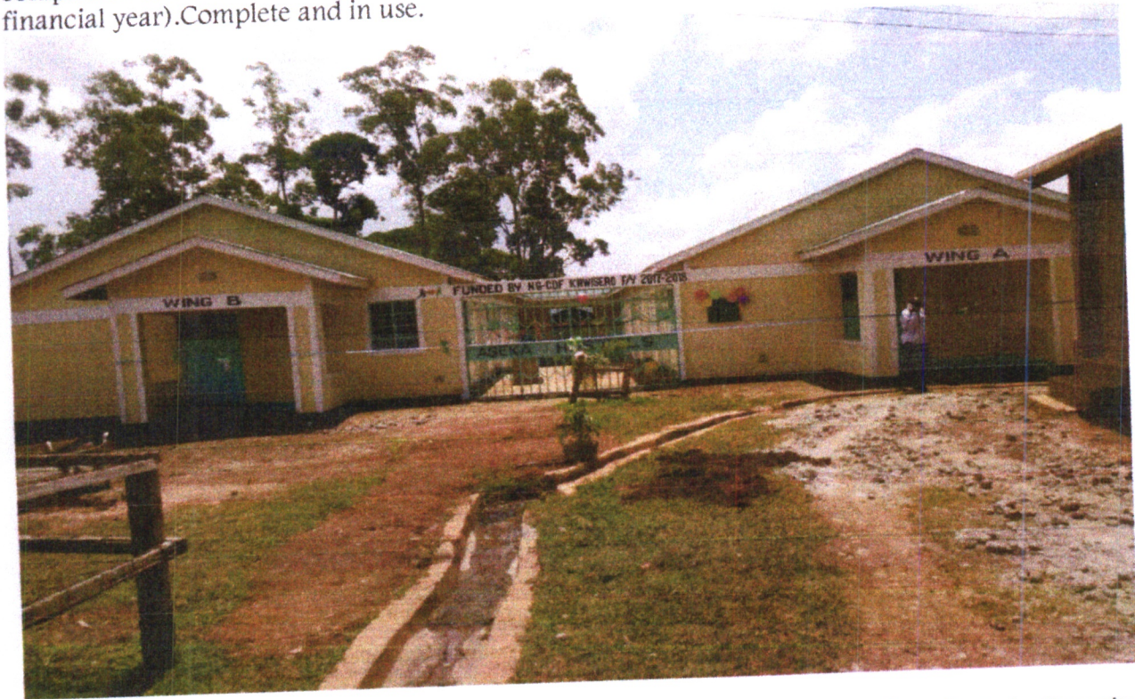
Emalindi Girls' Secondary School - Located in Kisa East Ward : Construction of a twin Dormitory.
