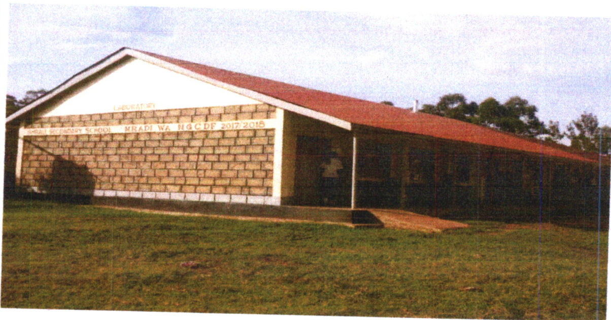
Shirali Secondary School - Located in Kisa Central Ward: Construction of a Single Science Laboratory. Funded in two financial years, 2017/2018 and completed under 2018/2019. In use.
