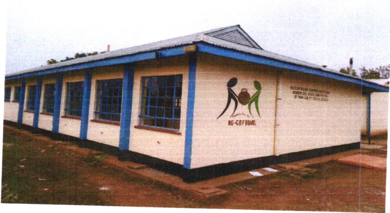
St. Mathew's Ikomero Secondary School - Located in Kisa West Ward: Construction of a Twin Science Laboratory. Funded in more than two financial years - completed under 2018/2019 following Presidential directive.
