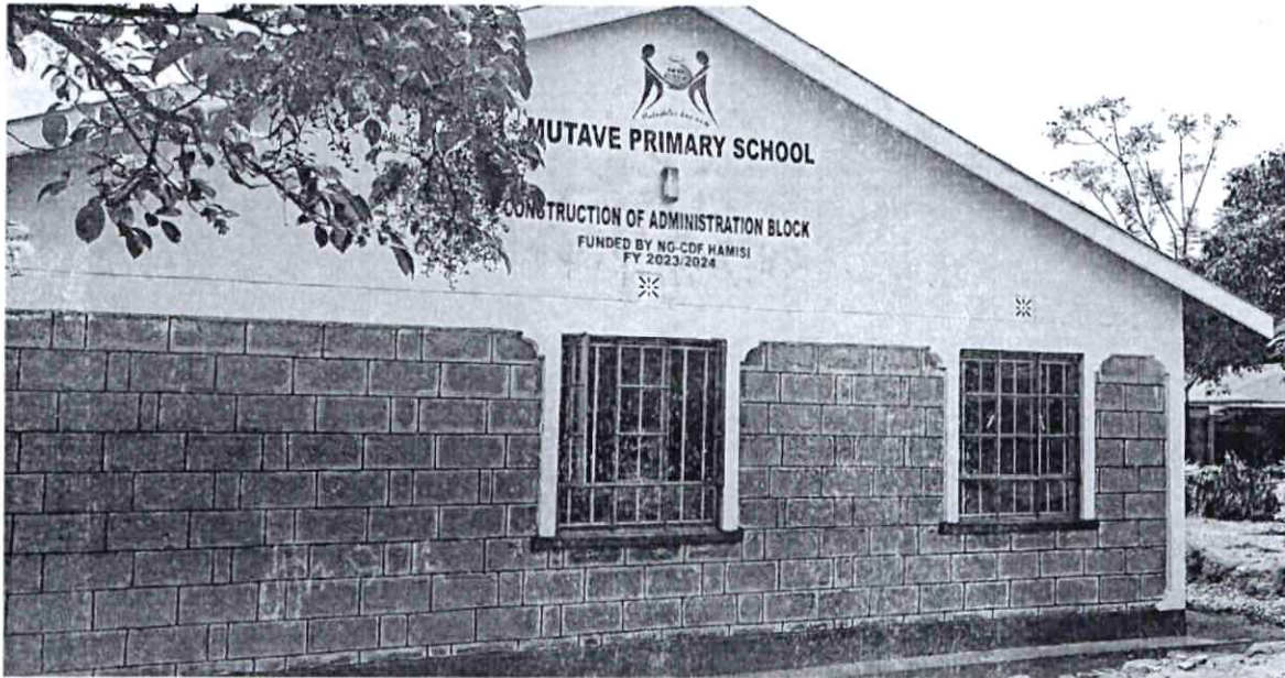
Fig. 2: Mutave Primary School newly constructed Administration block fully funded by Hamisi NG-CDF 2023-2024 Financial Year
