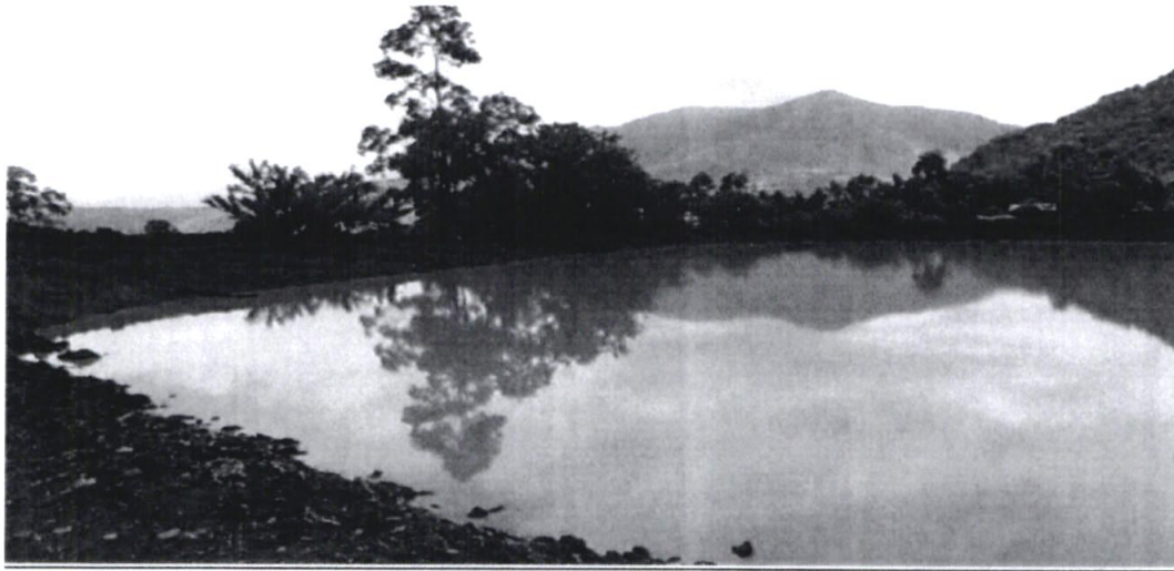
Sawe Pan in Elgeyo Marakwet County constructed under the National Rain Water Harvesting and Storage programme
