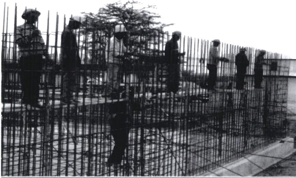
Construction of Narok Water Supply Project Treatment works
