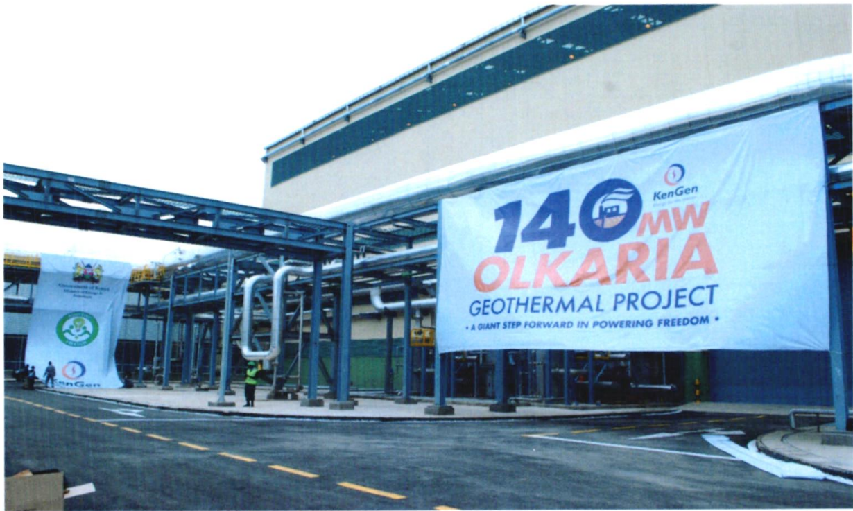
The Olkaria Geothermal Power Station – 140 MW Geothermal Project
