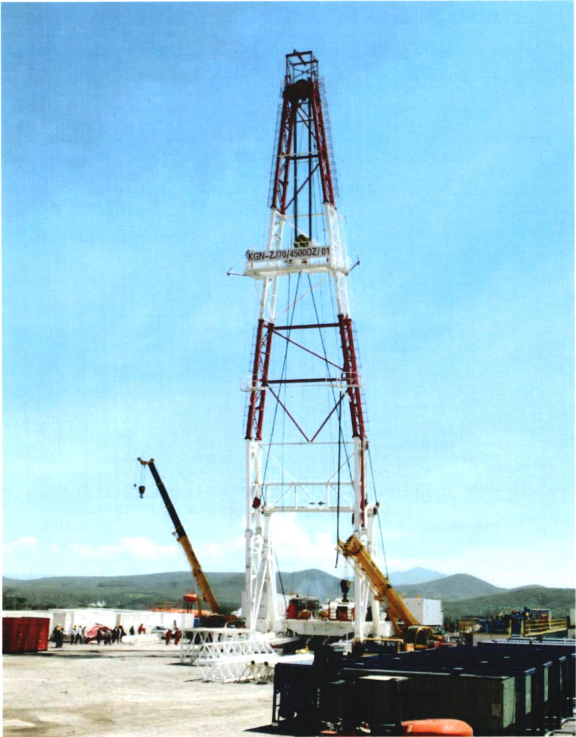
Drilling rigs at Olkaria Steam Field
