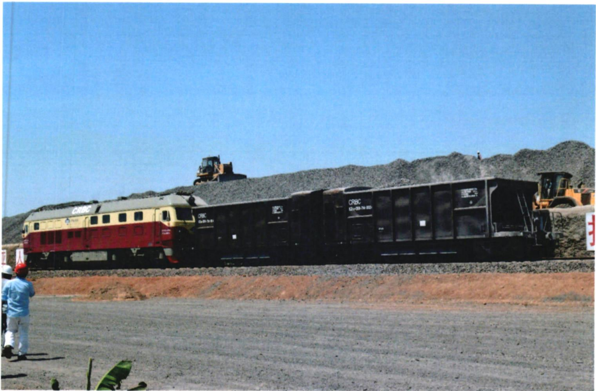
Locomotive Engine with wagon carriers at a construction site Construction of a typical bridge under SGR
