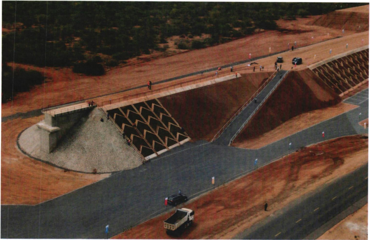
Construction of a typical bridge under SGR - In progress
