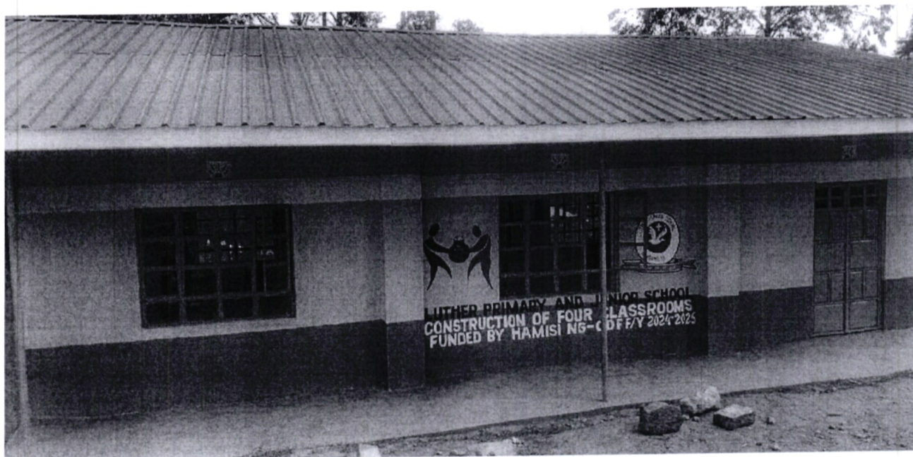
LUTHER PRIMARY SCHOOL - Construction of 4No. classrooms fully constructed by NG-CDF
