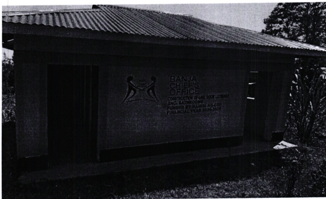
BANJA CHIEFS OFFICE –Construction of 6 door latrine and 2No. bathrooms
