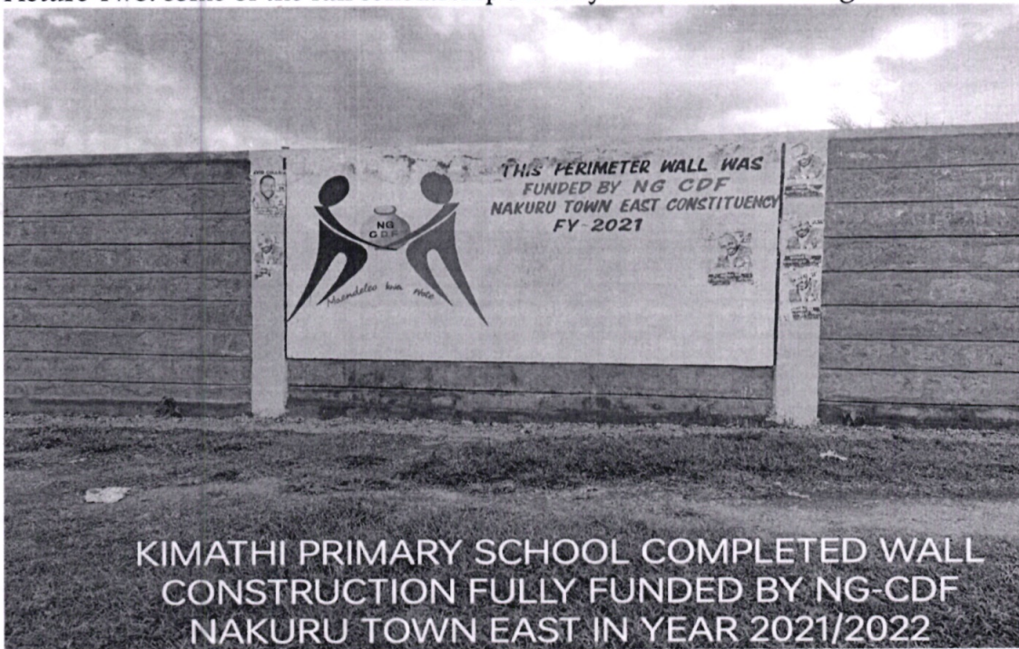
Picture Three: a perimeter wall constructed at Kimathi Primary School
