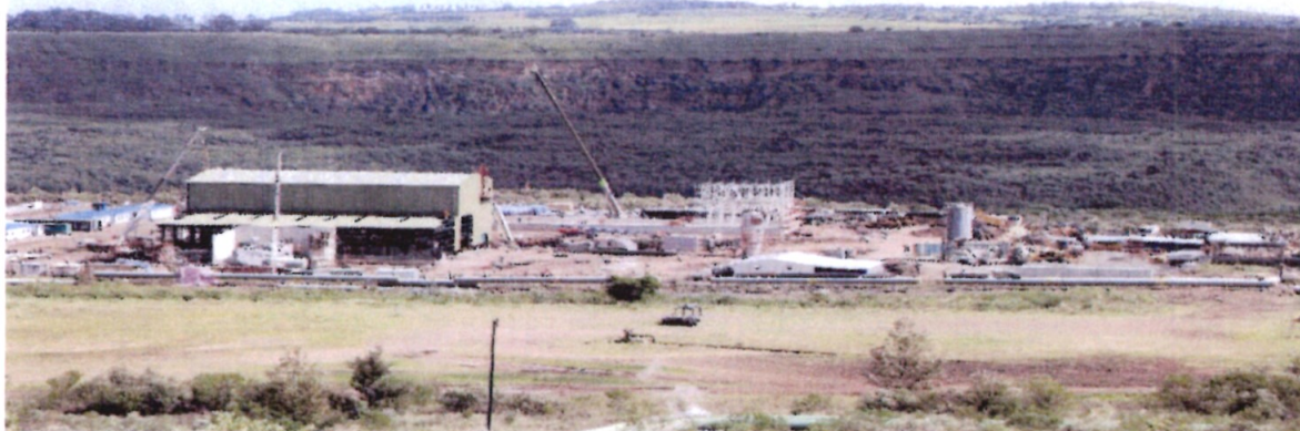
Globeleq Power plant as at June 2025
