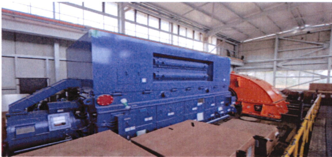
Unit3 turbine and generator erection is 60% completed.
