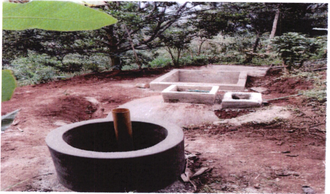
An ongoing construction of a domestic Biogas plant in Kakamega county by the State Department for Energy in the FY2024/25
