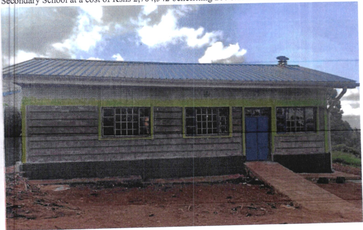
Figure 12: Completed kitchen for Kabebero Mixed Secondary School
