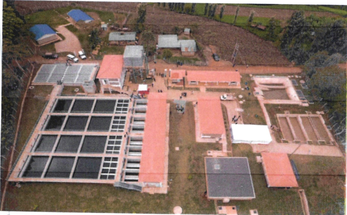
Figure 3: Completed Treatment Plant at Chogoria Water Infrastructure
