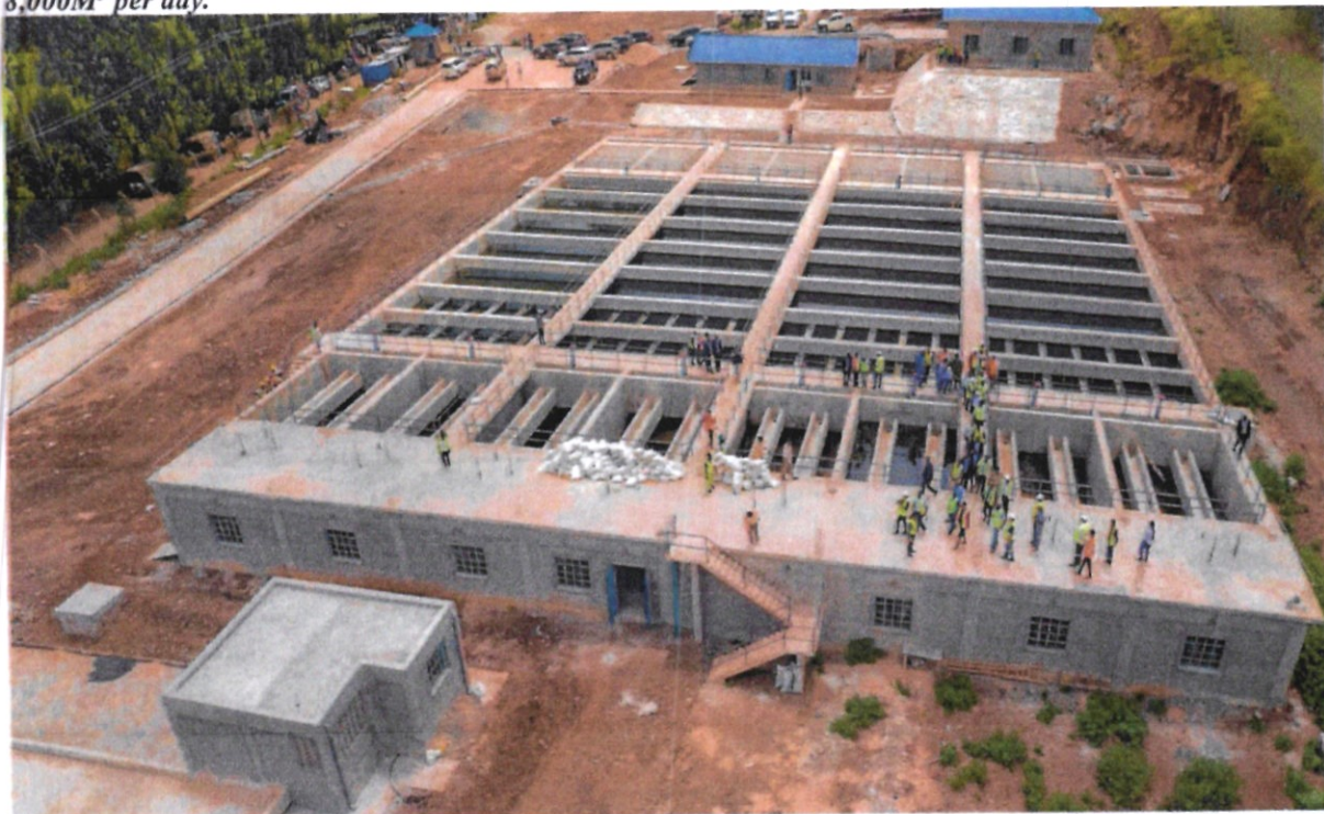
Figure 2: Ongoing works of the sedimentation basin at Muratiri Treatment Plant – Kerugoya-Kutus Water Supply Infrastructure within TWWDA area of jurisdiction. The treatment facility is supposed to treat 30,000m 3 /day of water.
