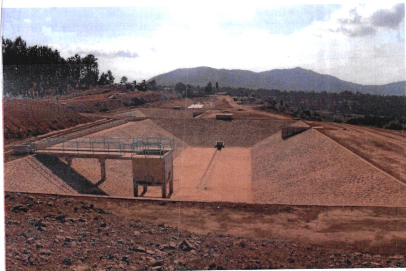
Figure 8: Anaerobic pond at Chogoria Sewerage Infrastructure
