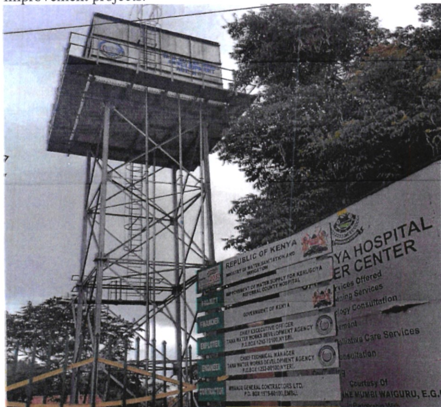
Figure 4: 48M3 steel Elevated tank at Kerugoya Referral Hospital
