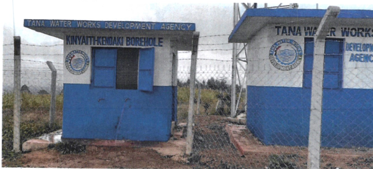
Figure 6: Pump house and water Kiosk at Kinyaiti-Kedaki Borehole with a yield of 54m 3 /day in Kieni, Nyeri County
