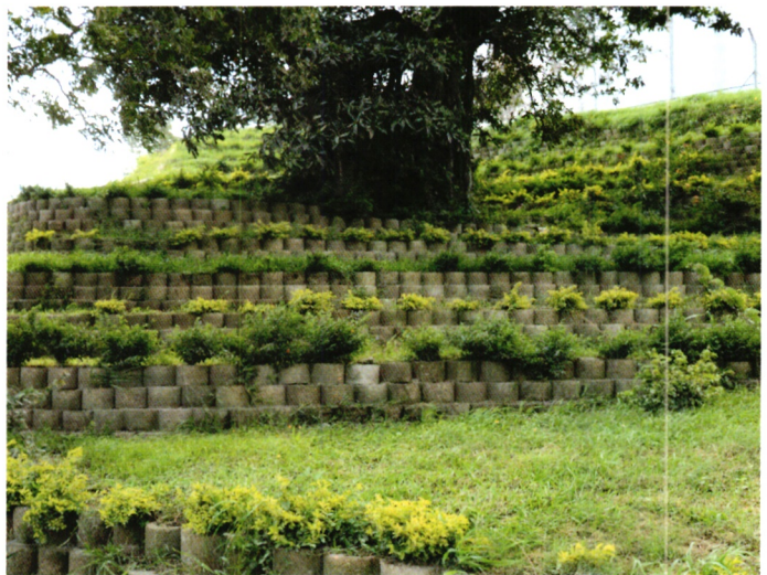
Site Progress Photos
