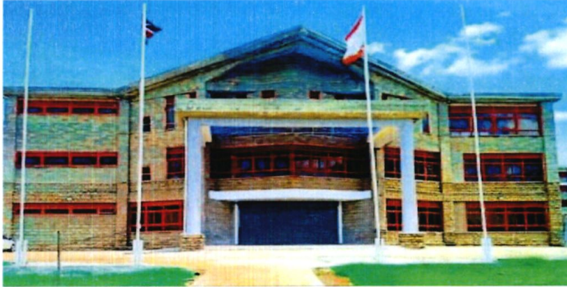
Ongoing construction of Library and Administration Block
