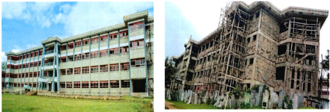
On-going Construction of Tuition Block A (Left) and B (Right)
