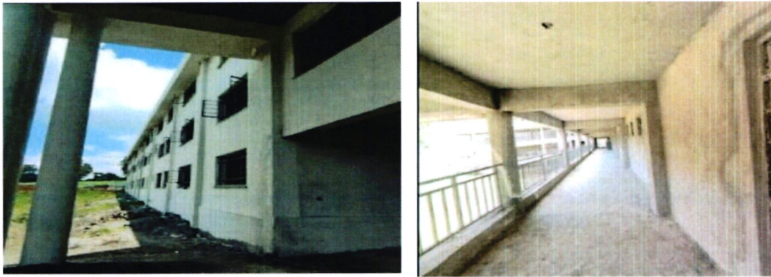
On-going Construction of Science Complex
