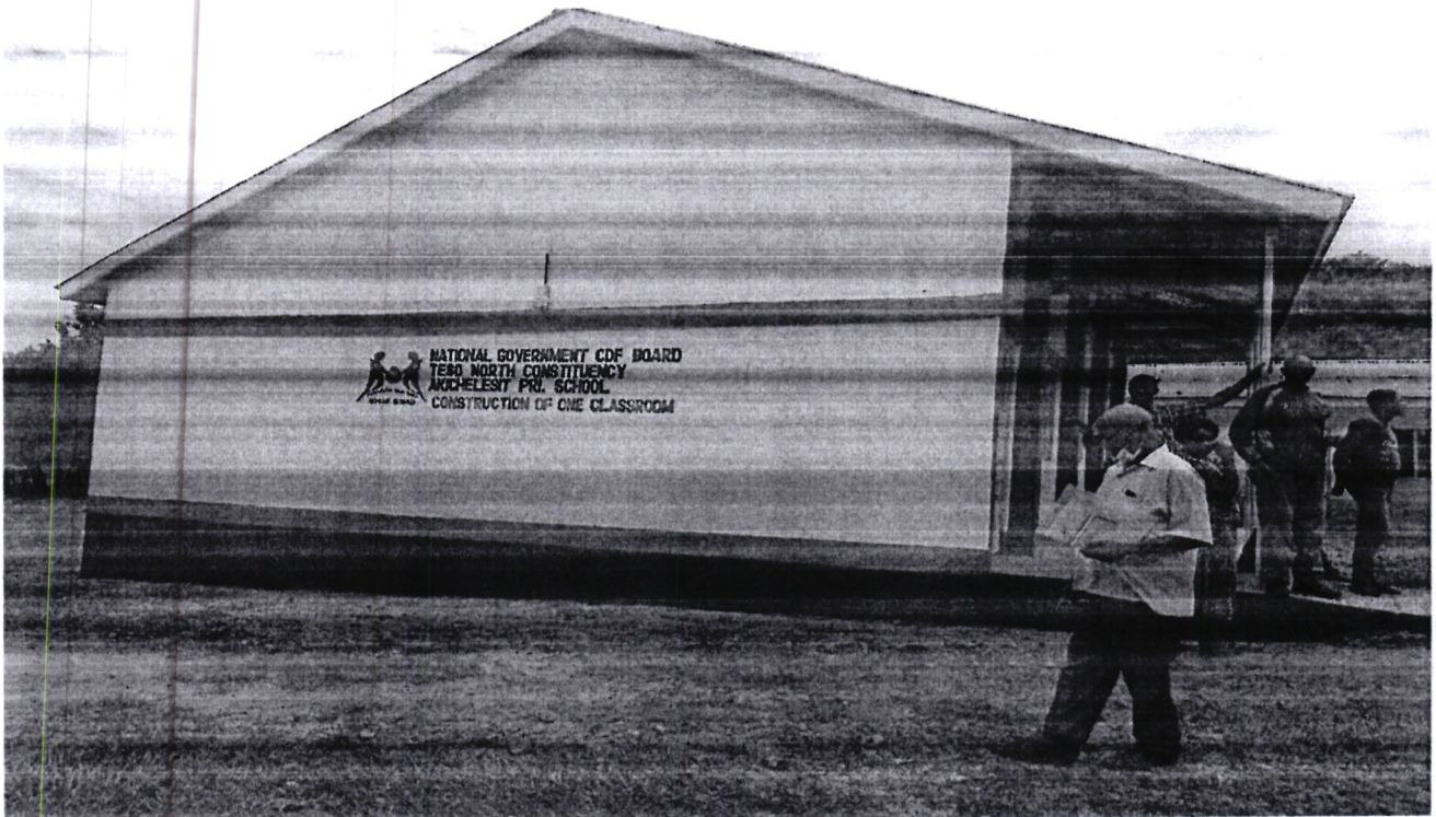
Akichelesit Primary School: Construction of one Classroom to Completion.
