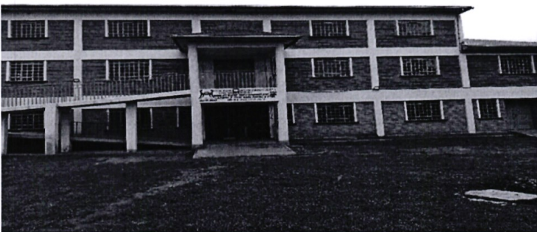
Marachi West ACC office constructed to completion
