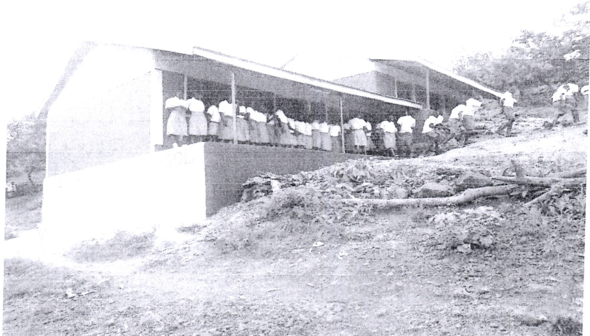
KUMBATHA PRIMARY SCHOOL- Completion of 2 class rooms Kshs. 400,000/=
