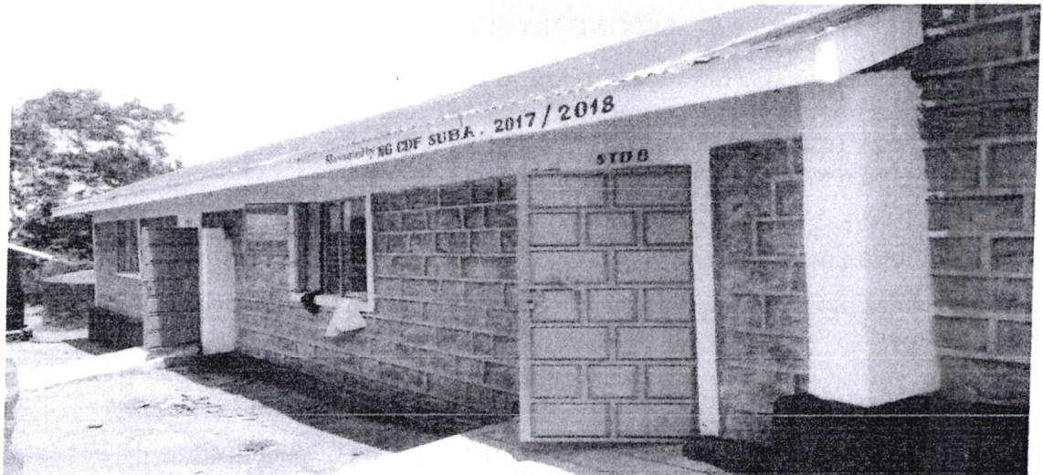
PUNDO PRIMARY SCHOOL- Renovation of 2 classrooms Kshs. 500,000/=
