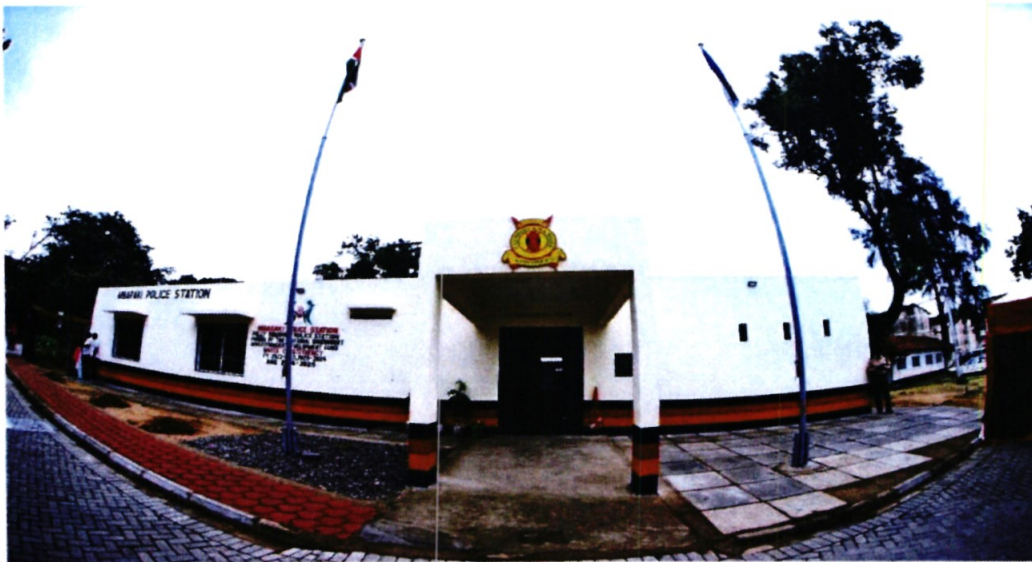
Figure 1.2 Refurbished Police Station
