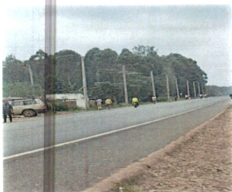
Street lights installed at Mosoch, Nyamira County
