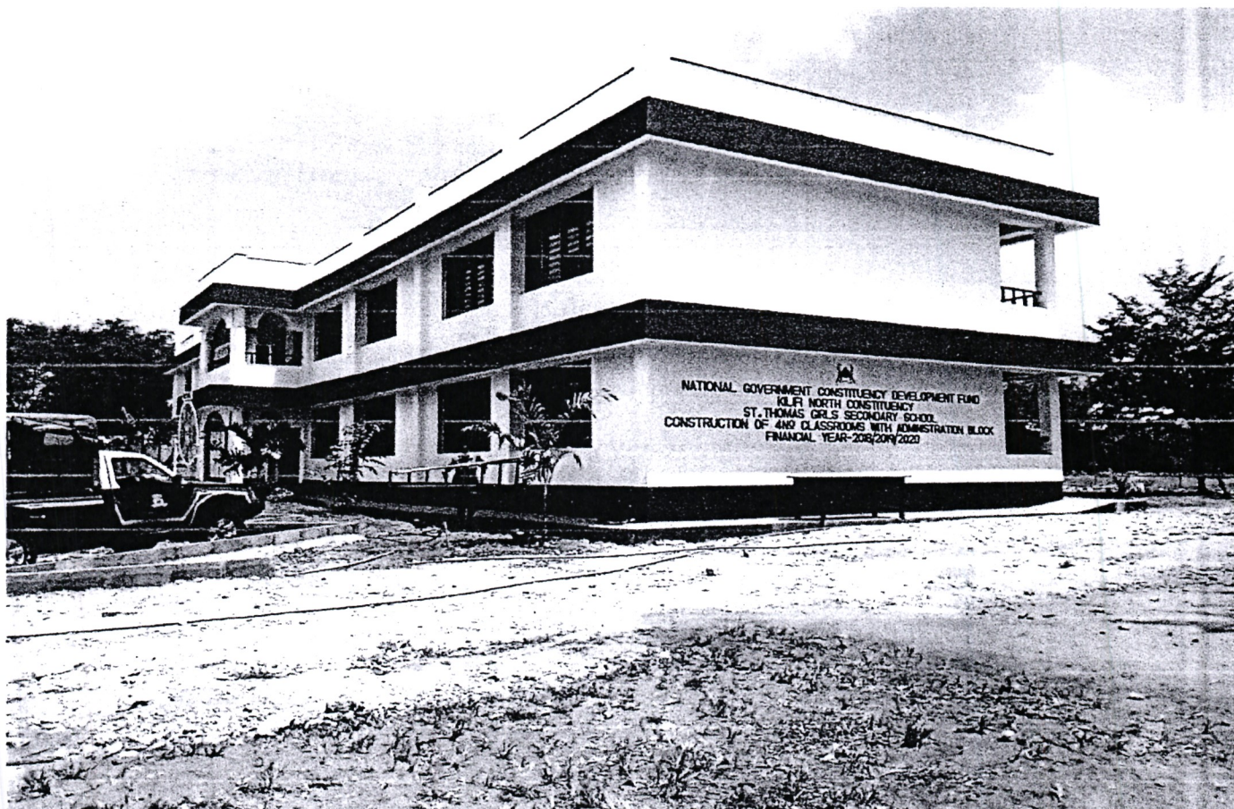
St.Thomas Girls secondary school- Four classrooms and an administration block
