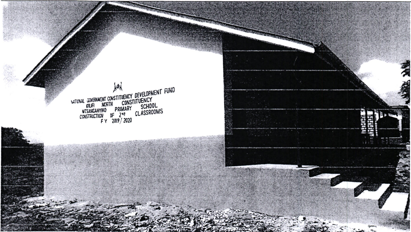
Mtsanganyiko Primary school- Construction of two classrooms
