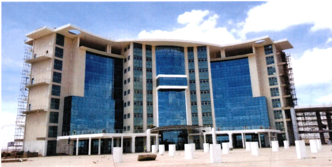
External view of Konza complex
