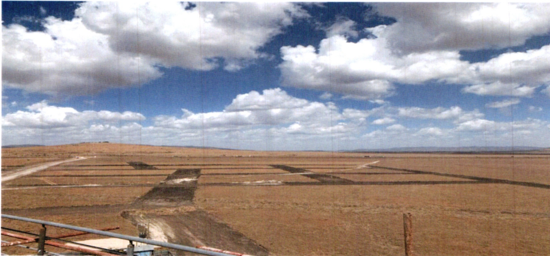
Aerial view of Access road under construction
