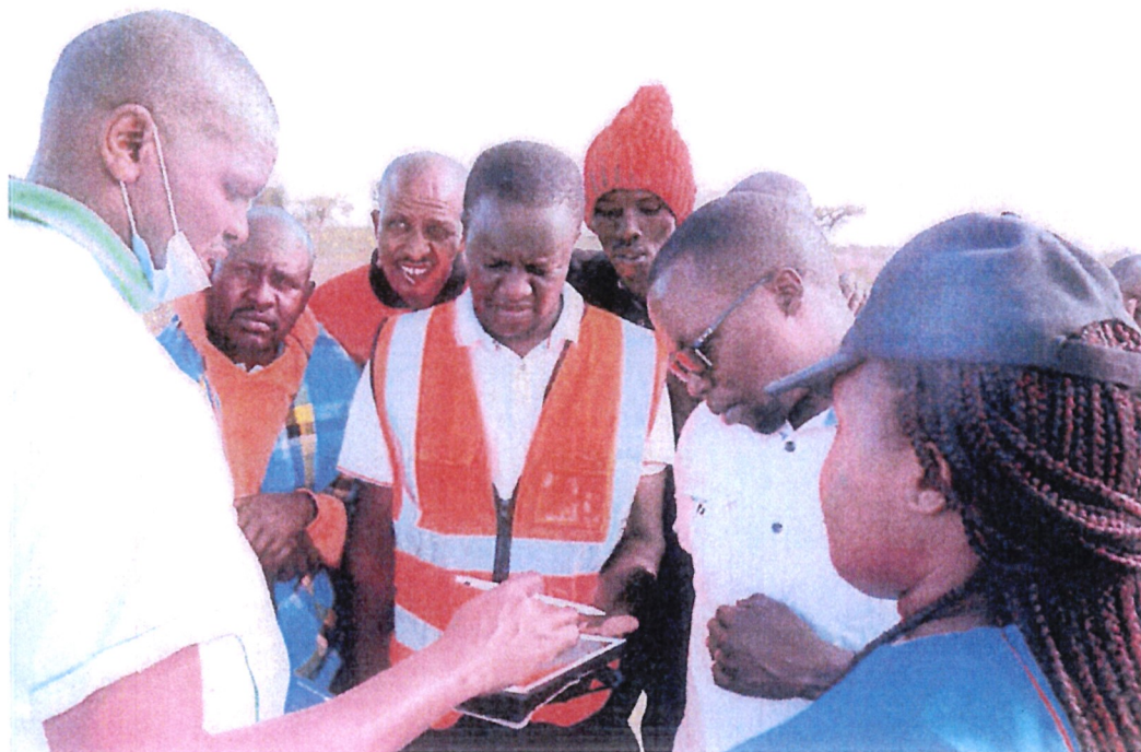
Eng. Ndiritu confers with Eng. Mathew (in orange reflector jacket) at the mini-grid installation site, as members of the community and SEED Coordinating team looks on.
