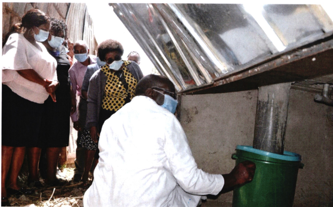
Dr. Messo explains how the fecal matter is collected from the UDDT facility at the school.
