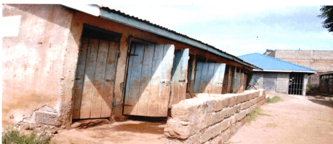
Left above, the old toilets versus the newly constructed sanitation facility (far right).
