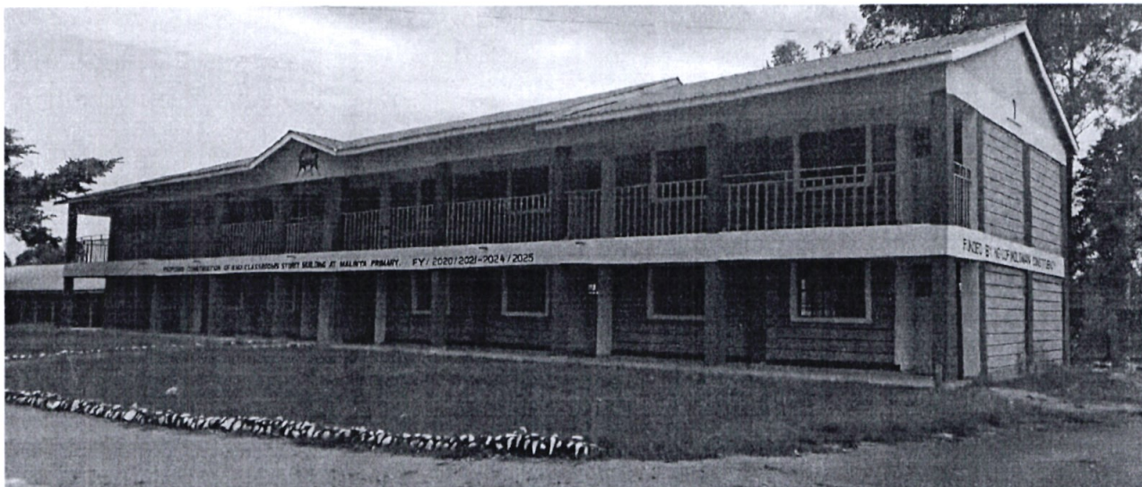
Malinya Primary School-Construction of 8 No storey Classrooms
