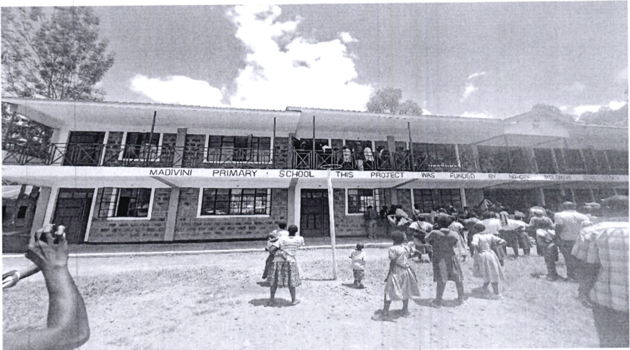
Madivini Primary School-Construction of 8 No Storey Classrooms
