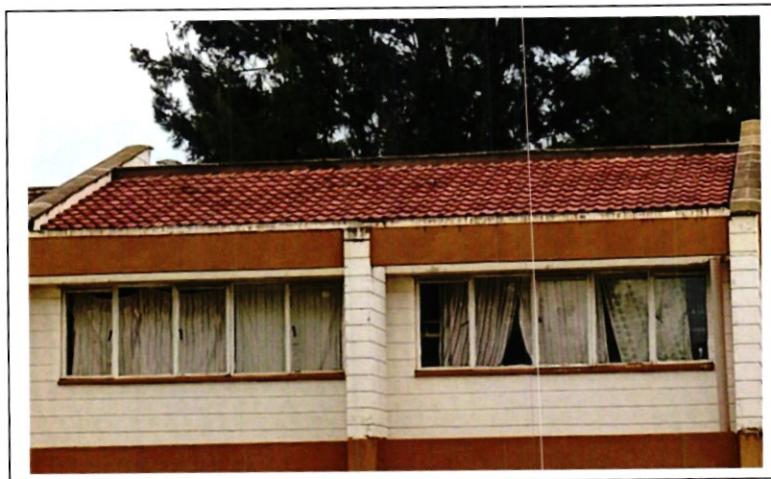
Figure 17: Repaired Hostel Roof
