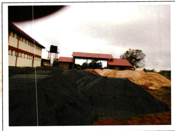
Figure 18b: Block Making Materials
