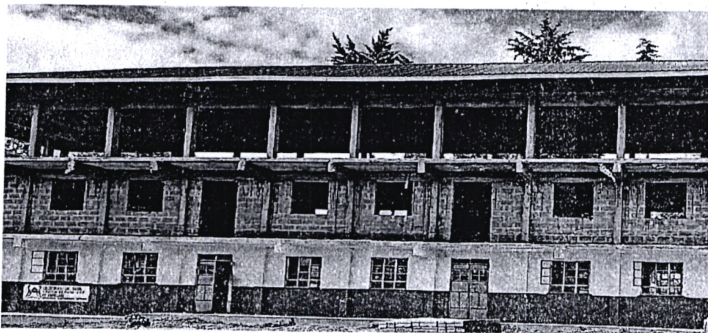
MASANA SECONDARY SCHOOL. CONSTRUCTION OF TUITION AND ADMIN BLOCK
