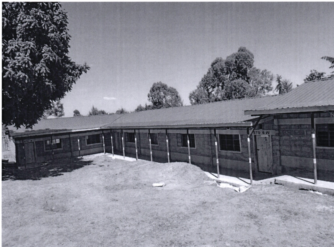
Kapchila secondary school building of 4 classrooms.
