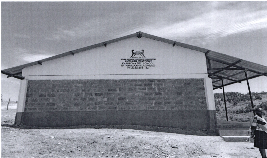
Kapkecha secondary school construction of 4 classrooms to completion
