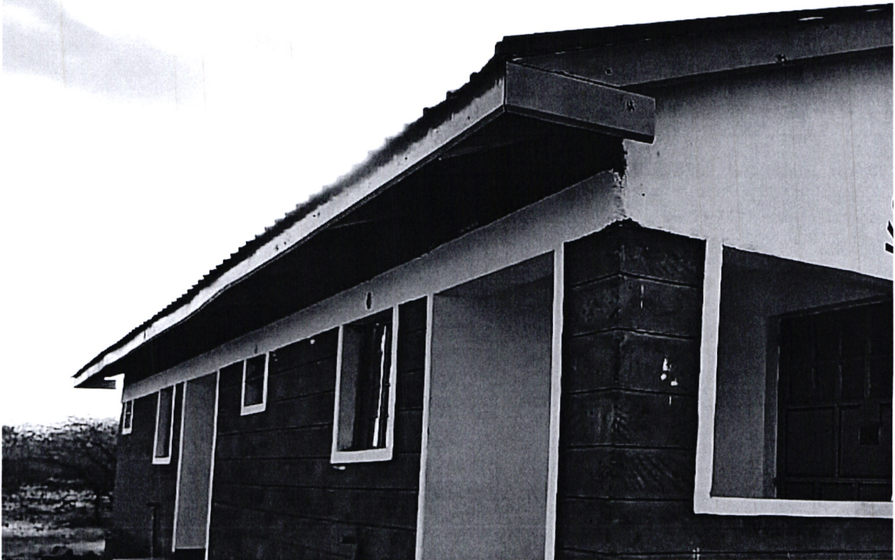
COMPLETED KOMIYA PRIMARY SCHOOL STAFF HOUSES FUNDED BY NGCDF KAJIADO WEST 2018/19
