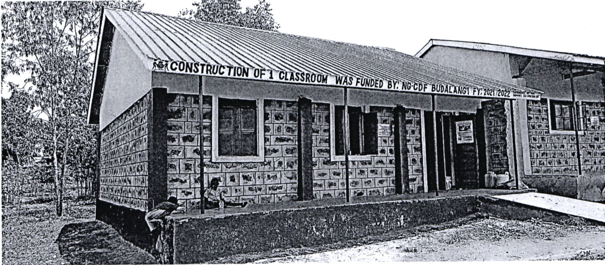
Construction of one (1No.) new classroom to completion at Munani primary school FY – 2021/2022
